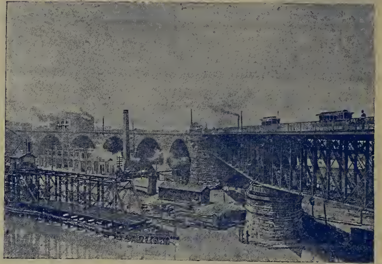
SUPERIOR STREET VIADUCT, CLEVELAND.
