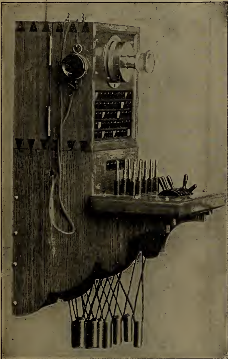
FIG. 2—WESTERN TELEPHONE CONSTRUCTION CO.'S SWITCHBOARD.
