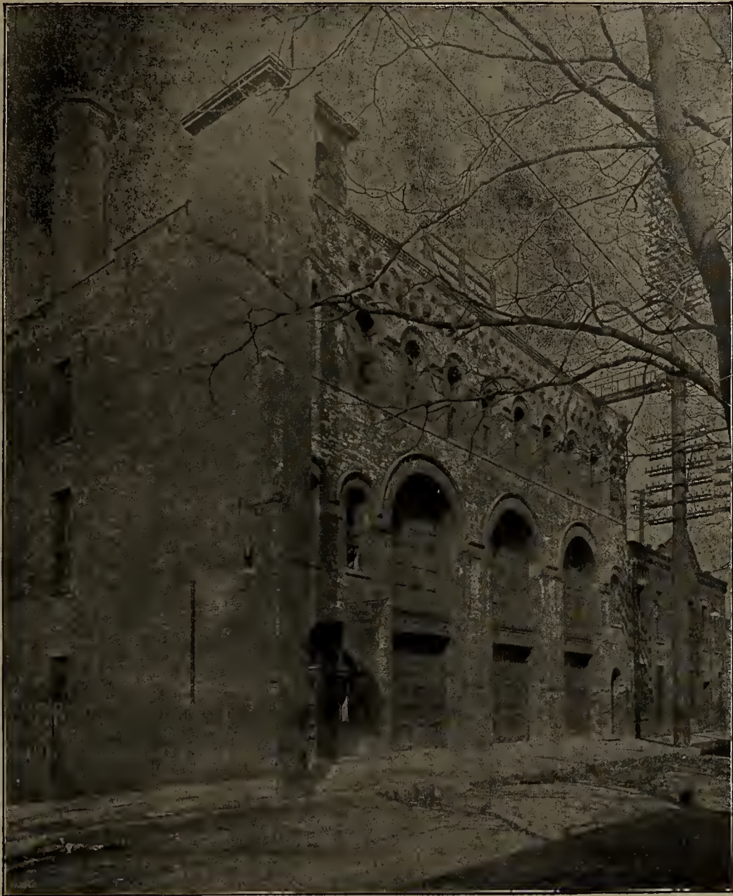
STATION OF CITIZENS' ELECTRIC ILLUMINATING CO., BROOKLYN.
