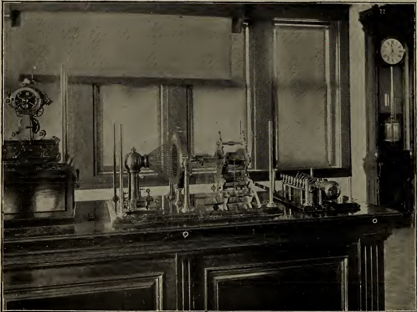
FIG. 3—AUTOMATIC LINE TESTER AND DIAL TRANSMITTER, BROOKLYN FIRE ALARM HEADQUARTERS.
