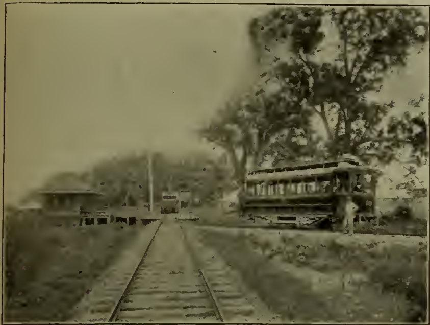
BACK RIVER STATION MONTREAL PARK AND ISLAND RAILWAY.
