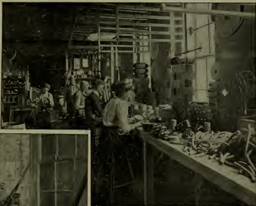
FIGS. 4 AND 5.—MAKING COUPLINGS, ELBOWS, JOINTS, ETC.
