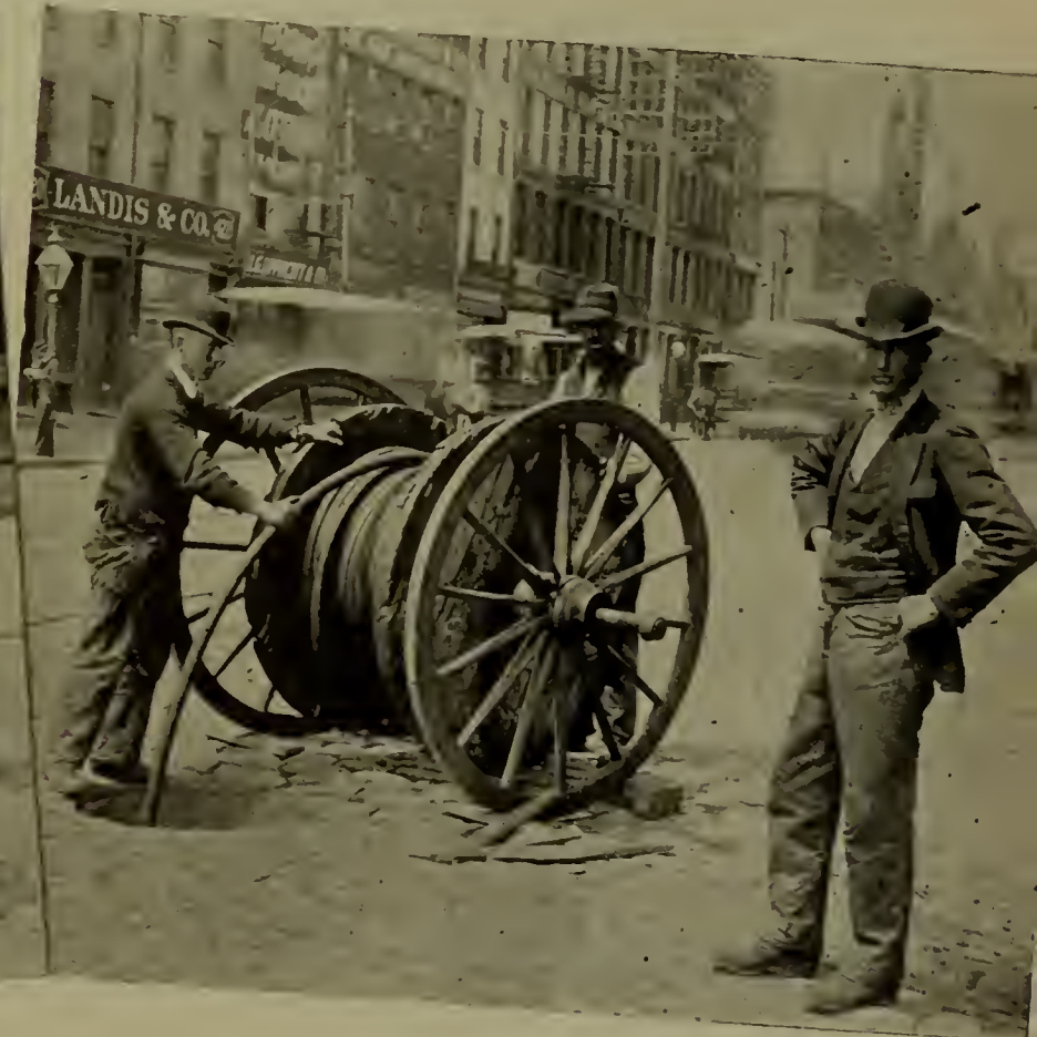
DRAWING IN UNDERGROUND CABLES, PHILADELPHIA TRACTION CO.
