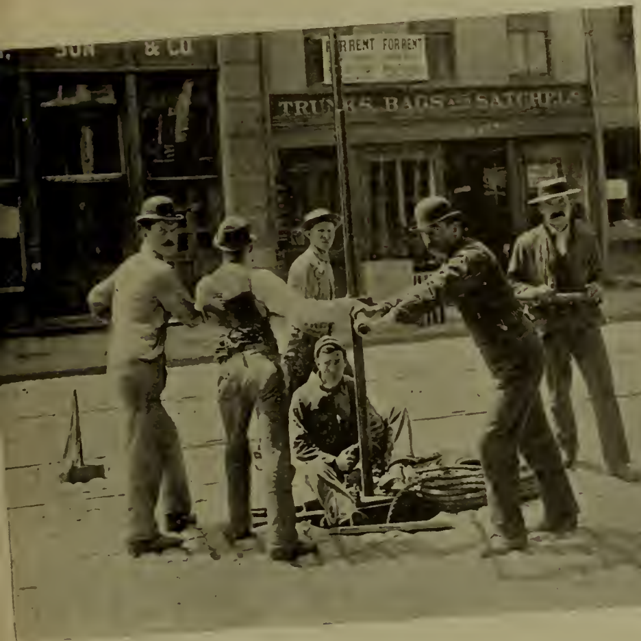
DRAWING IN UNDERGROUND CABLES, PHILADELPHIA TRACTION CO.
