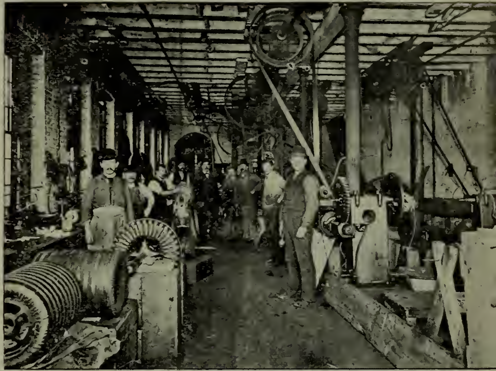
SECTION OF MAIN FLOOR, DYNAMO, COMMUTATOR AND ARMATURE DEPARTMENT, STUCKY & HECK ELEC. MFG. CO.
