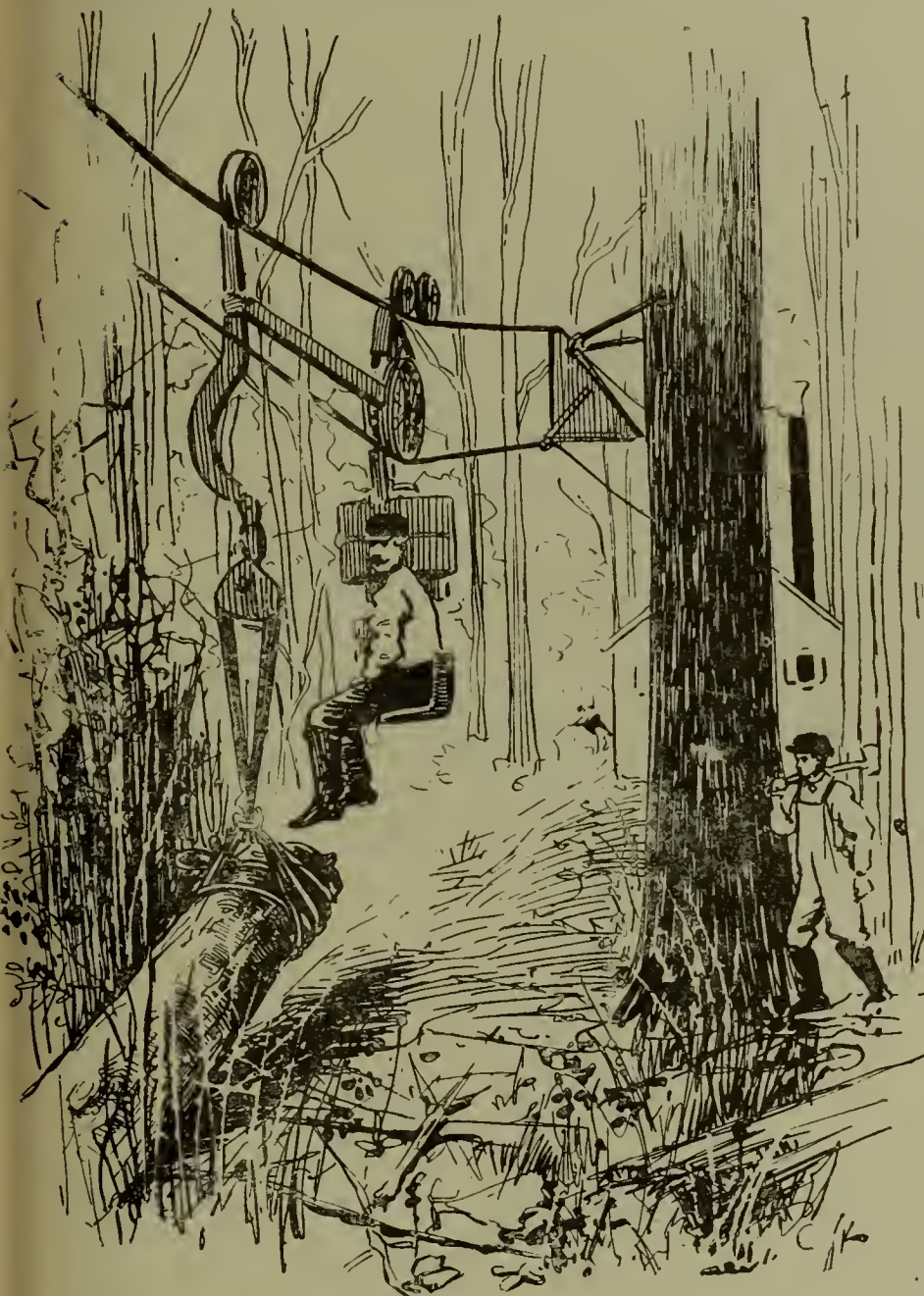
LOG HAULING BY ELECTRIC POWER.
