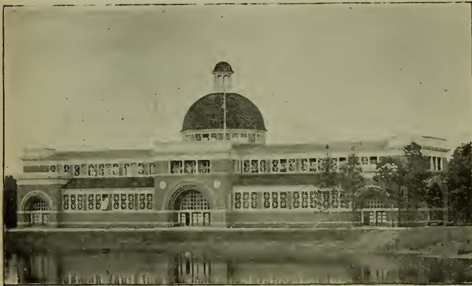
ELECTRICAL BUILDING, ATLANTA EXPOSITION.
