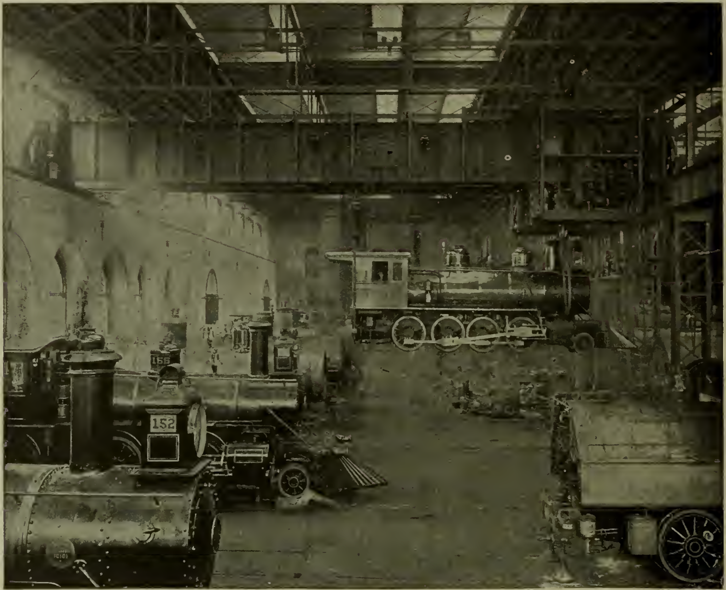
100-TON SELLER'S CRANE AT BALDWIN LOCOMOTIVE WORKS.
