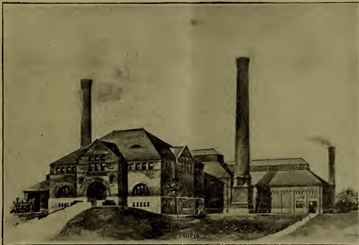
The Ridgewood Pumping Station of the Brooklyn Waterworks.
