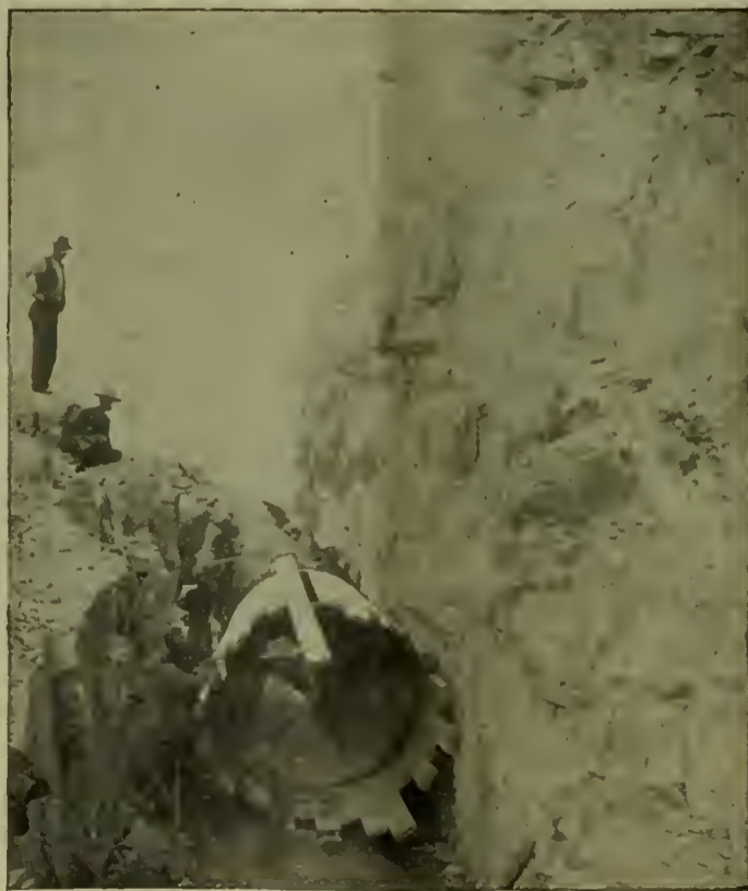
Fig. 2.—Making Wooden Pipe.
