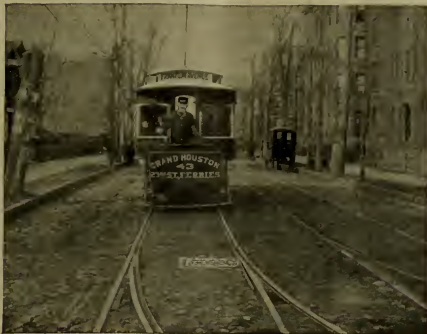
Surface View of Automatic Electric Switch. New York Switch & Crossing Co.
