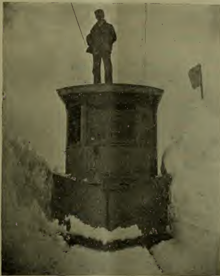
Removing Snow at Skowhegan, Maine.
