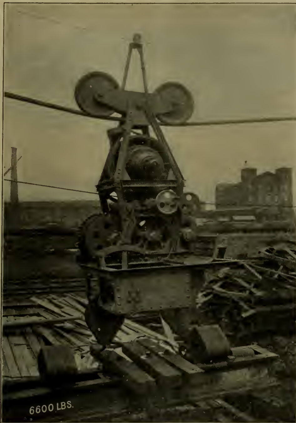
Fig. 7.—Loaded Crane on Cable.
