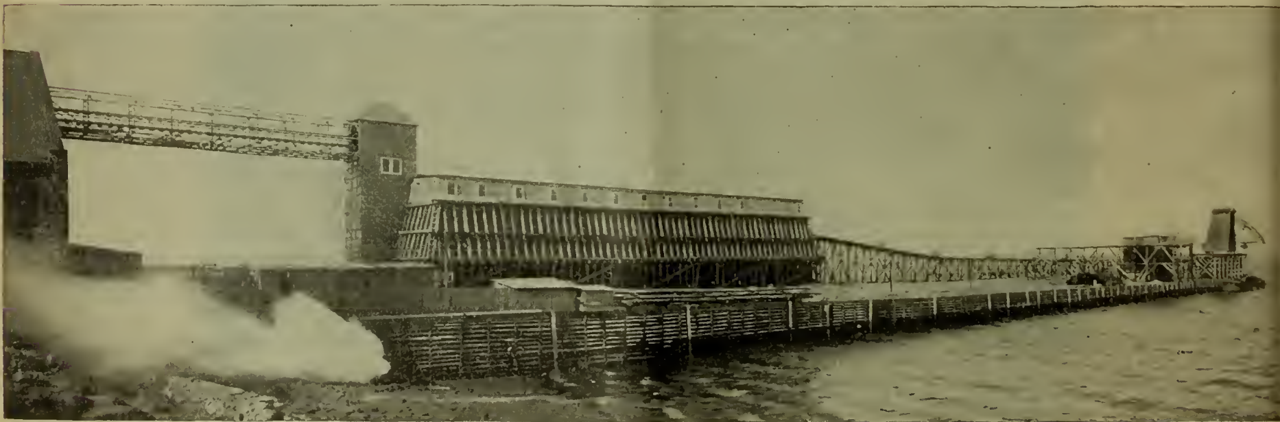
General View of the Steam Shovel, Cable Railway and Conveyor at the Southern Power Station of the Brooklyn Heights Railroad Company.
