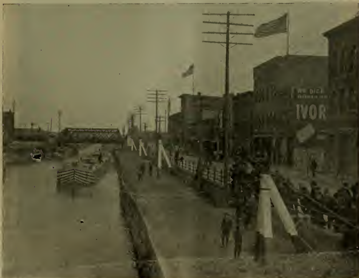
Fig. 5.—Test on Erie Canal at Tonawanda, N. Y.
