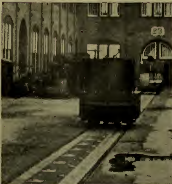
G. E. Surface Contact System, Showing Stretch of Track in Yards of General Electric Company's Works at Schenectady, N. Y.
