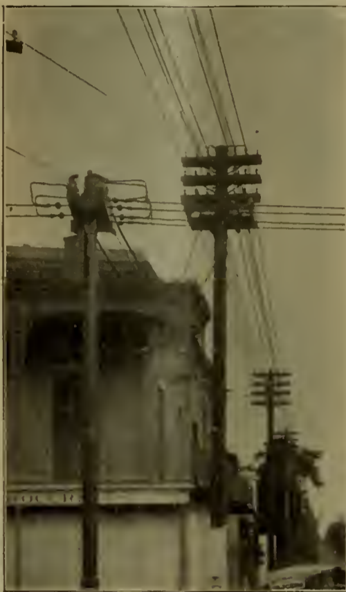
Fig. 1. Sectional Feeding Point.
