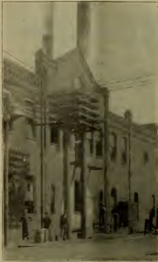
Anchor and Terminal Poles at Power Station.
