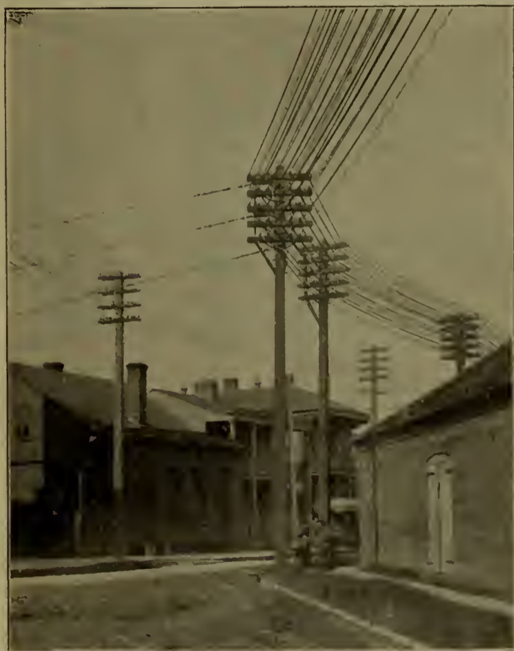
Feed Line Construction at Curve in Street.
