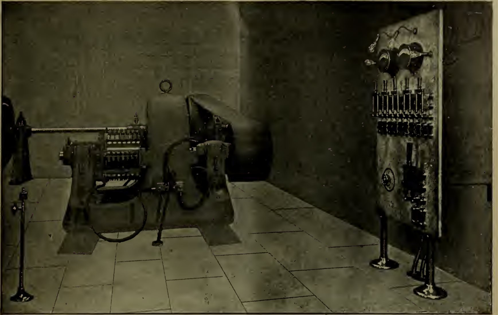
100 K. W. Belted Generator, Plant of the Lane & Bodley, Cincinnati, O. (Triumph Elec. Co.)
