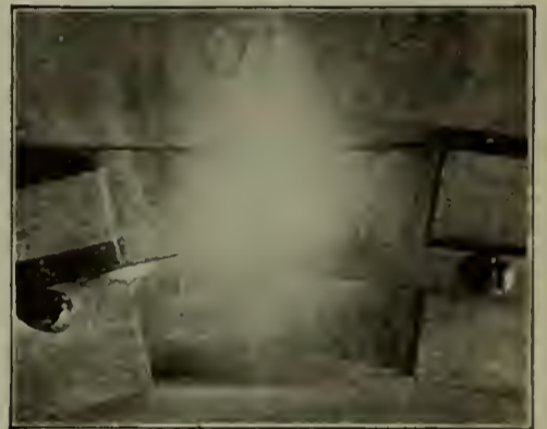
Terminals Supporting an Arc.
