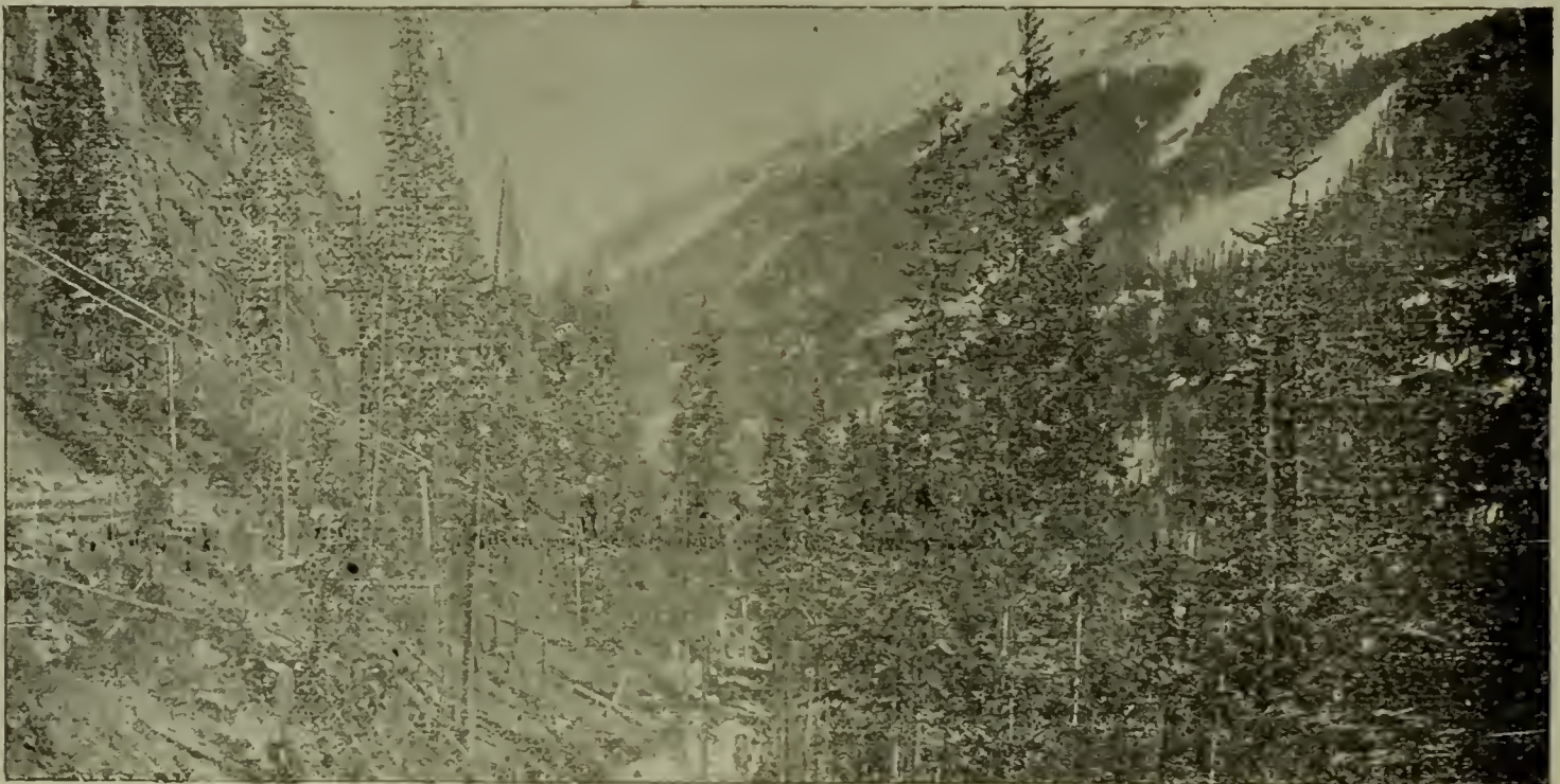
Transmission Line, "Virginius" Mine, Rising Up the Mountain Side.
