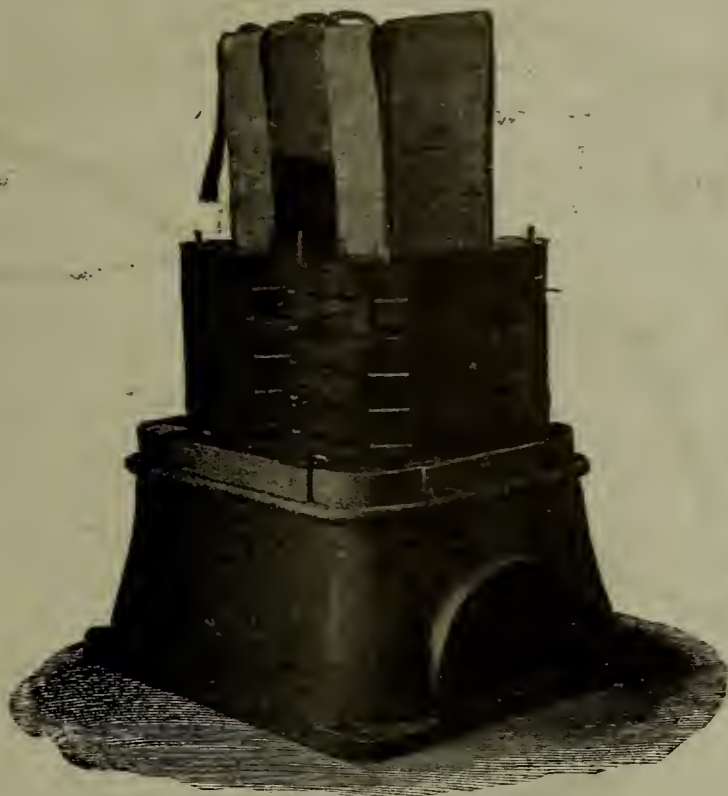
Construction of Air Blast Transformer.
