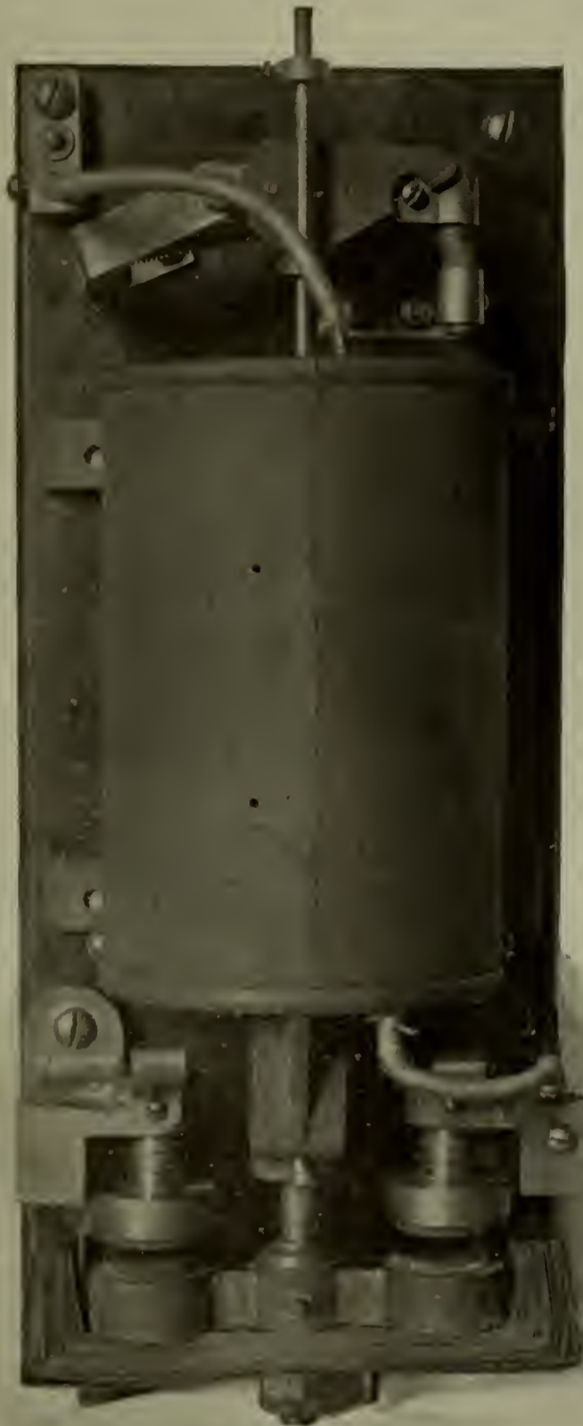
Complete Vault Switch.
