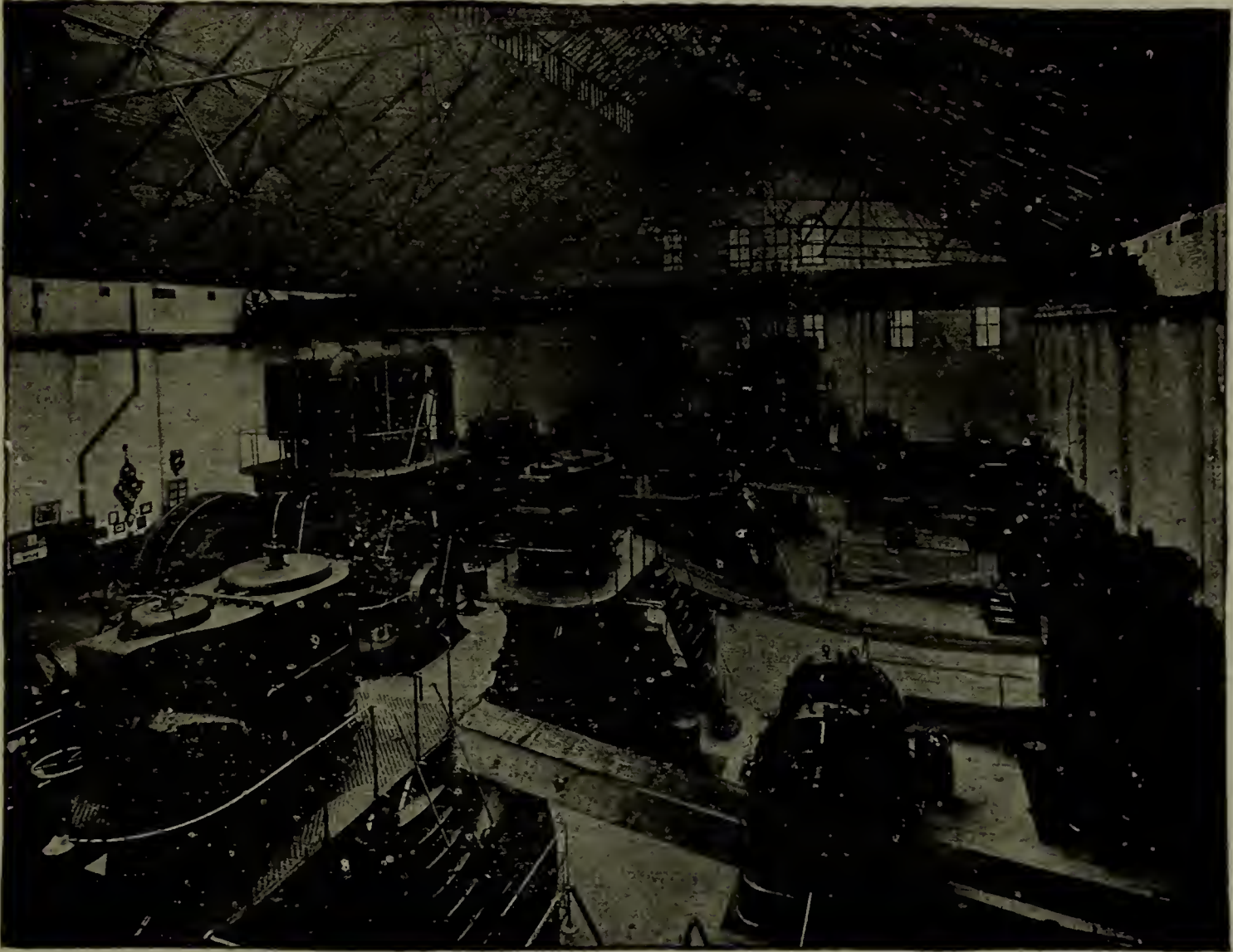
Station Equipment for Large Street Railway and Power Plant.
