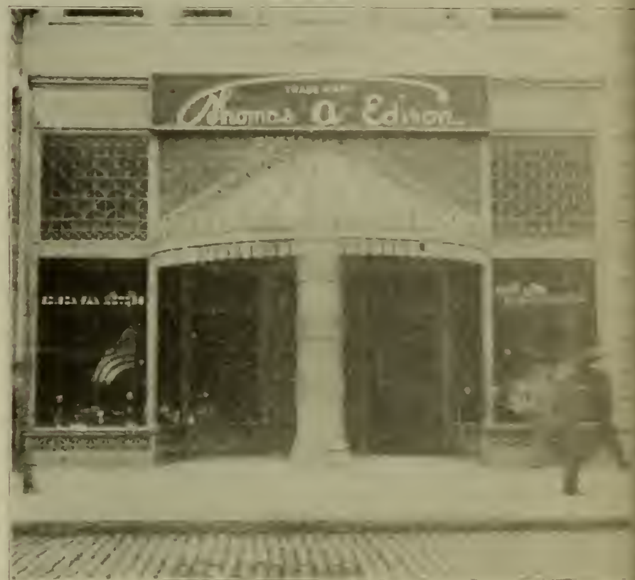
A Conspicuous Example of "Flush Letter" Type of Sign Construction.
