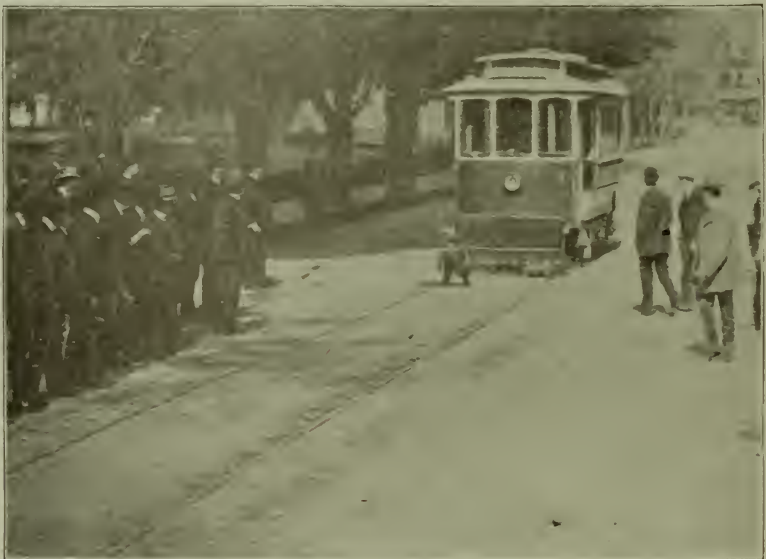
Fender Dropped to the Ground.
