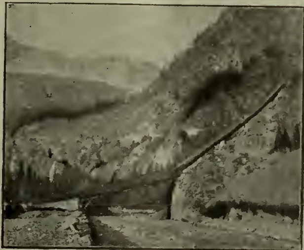
Electrolytic Chlorate.—Pipe Lines on Bridge.
