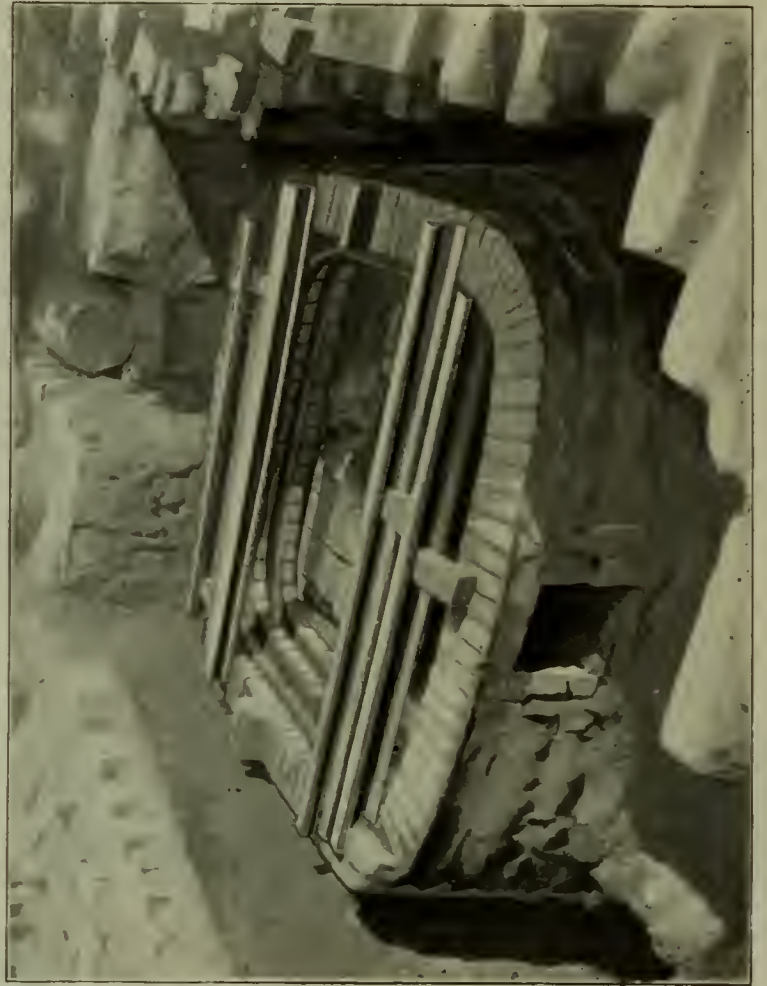
1 and 2, Illustrate Laying of 1st Course of Rails and Bricks.
