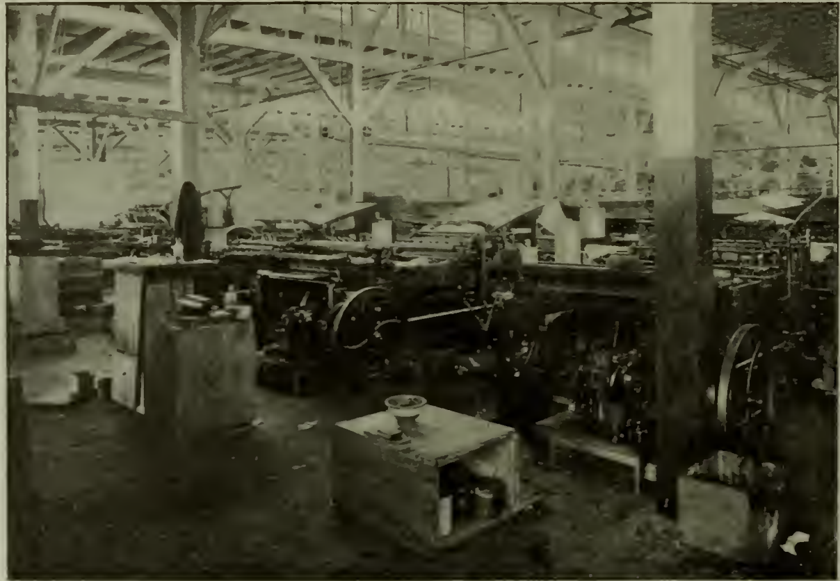
Printing Room Showing Electrically Driven Presses and Absence of Belting and Shafting; 45 C. W. Motors Installed in This Room.
