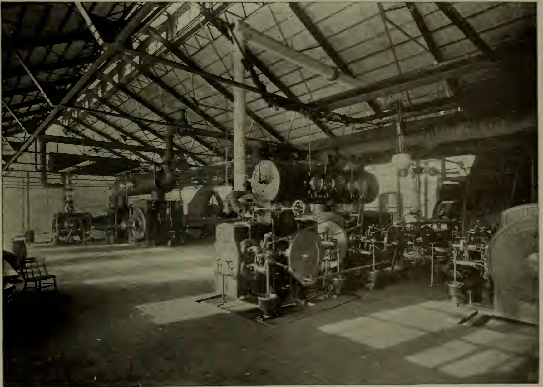
The Steam Plant of a Power Station.
