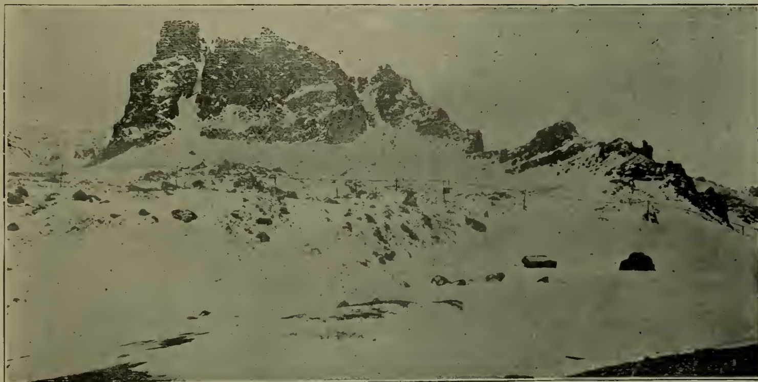
Transmission Line In the Rockies.
