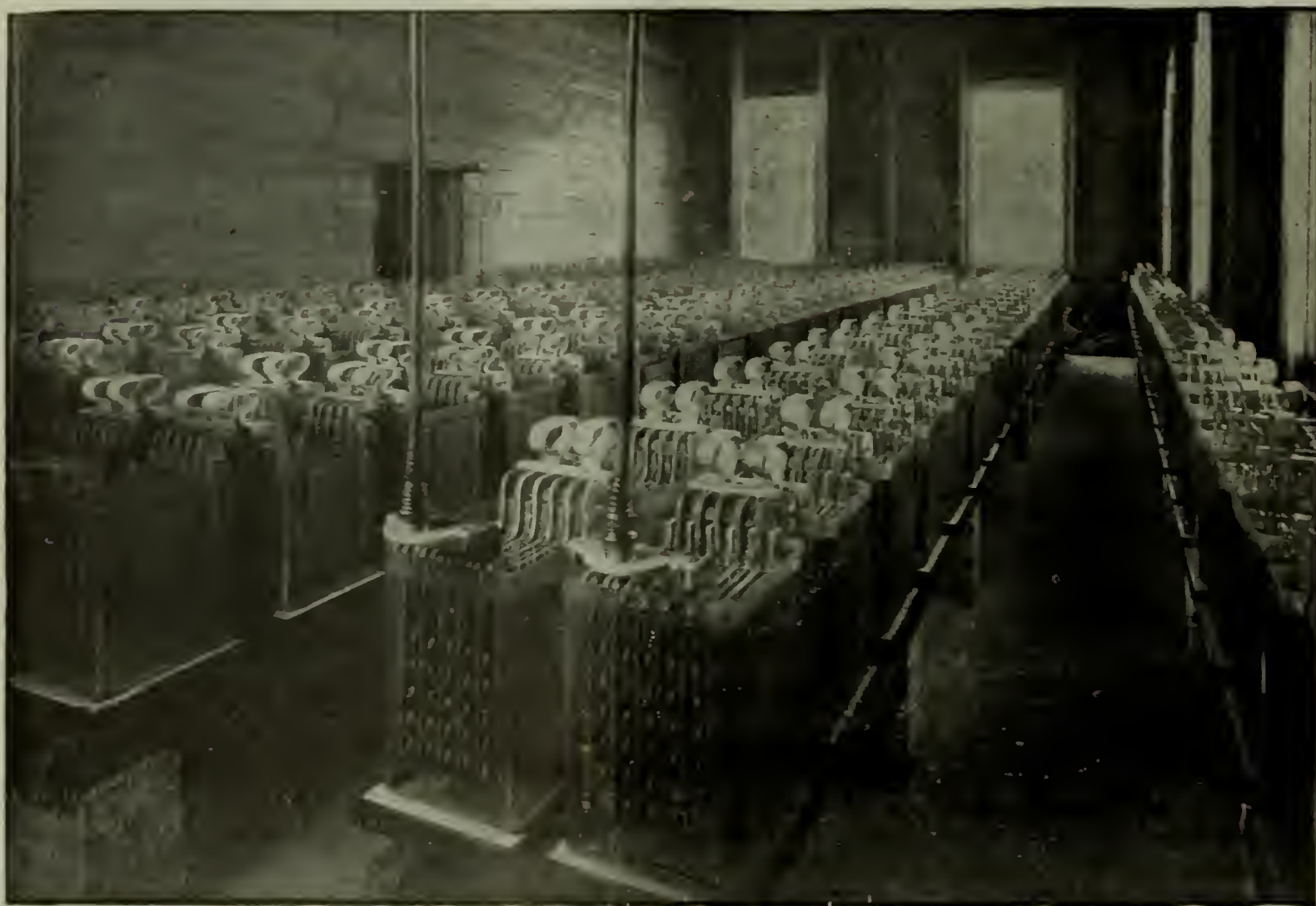
Storage battery plant.
