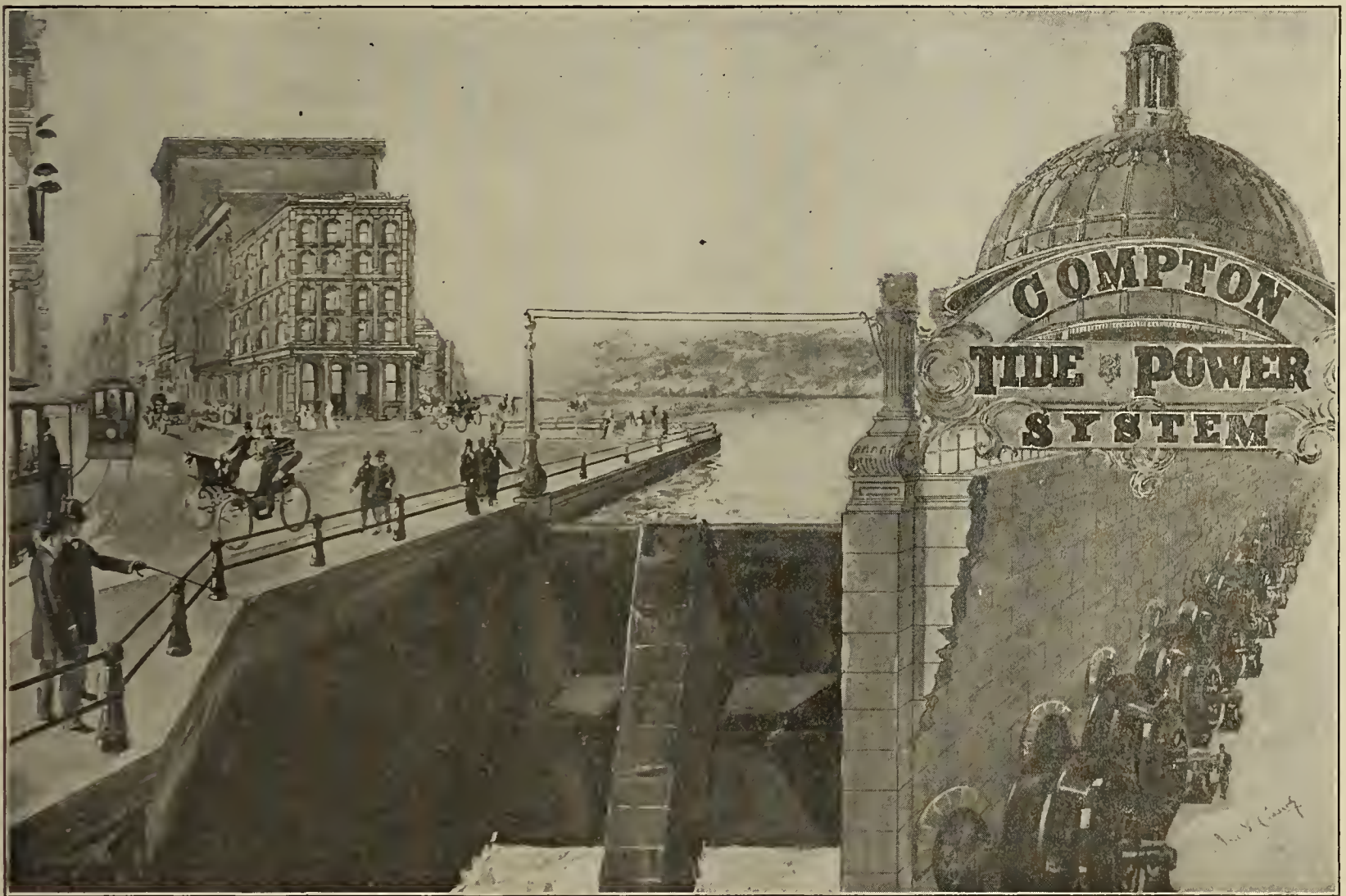
Interior of Power House. Compton Tide Power System.
