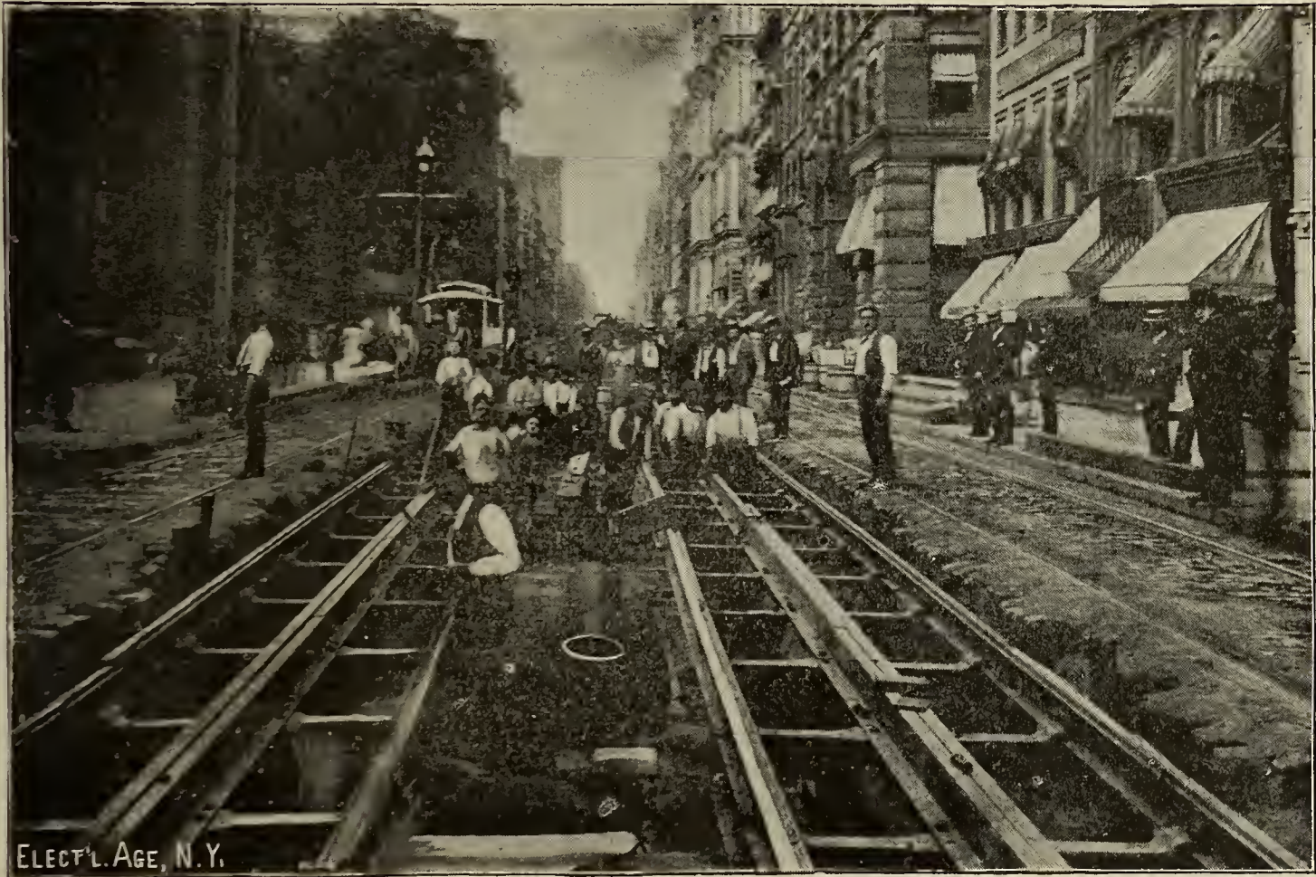
Re-Constructing for Underground Trolley.
