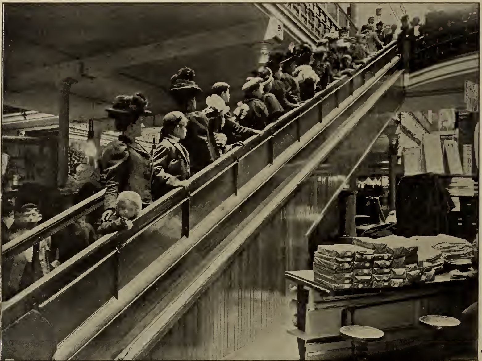
Reno Inclined Elevator Installed in Department Store.
