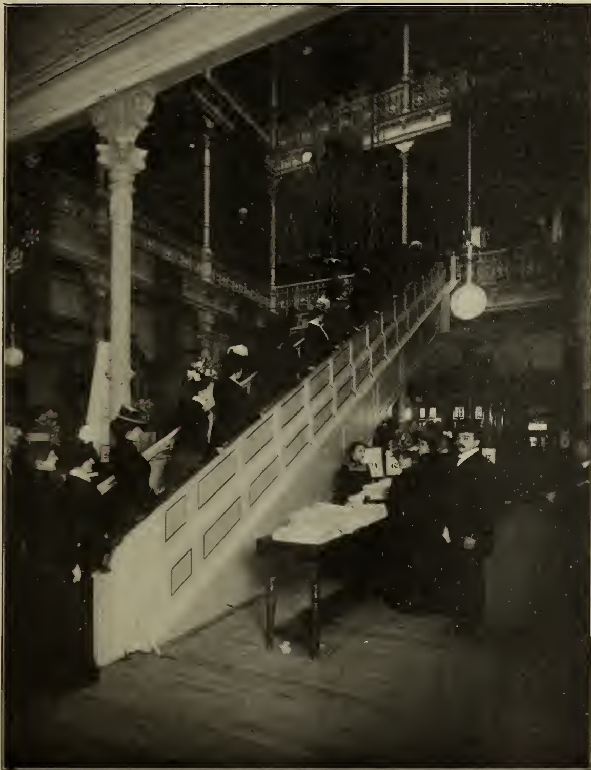
Elevator Installed in Bloomingdale Brothers, 59th Street & 3d Avenue, New York.
