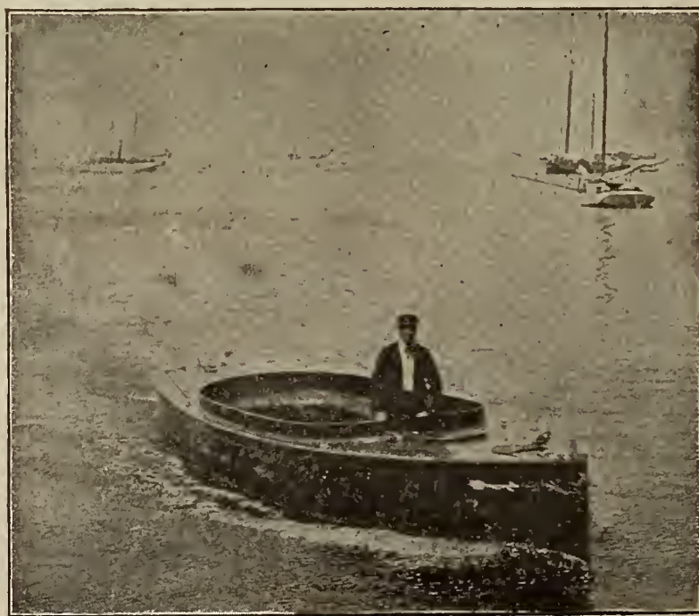
An Electrically Propelled Launch. Power Delivered by Storage Batteries.
