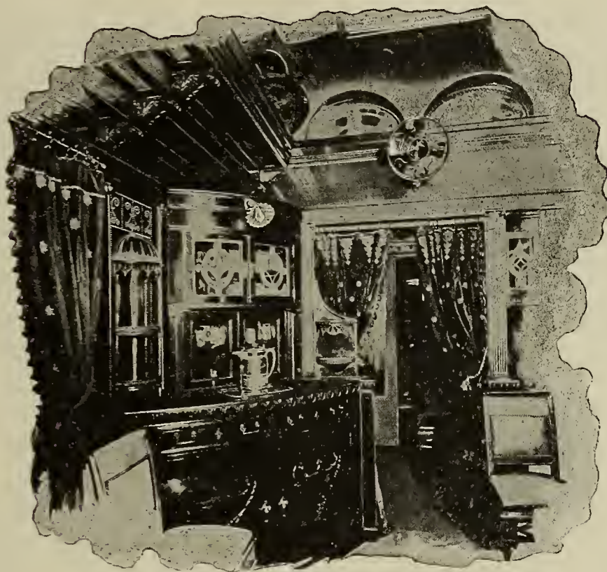
Electric Lights and Fan in Buffet.
