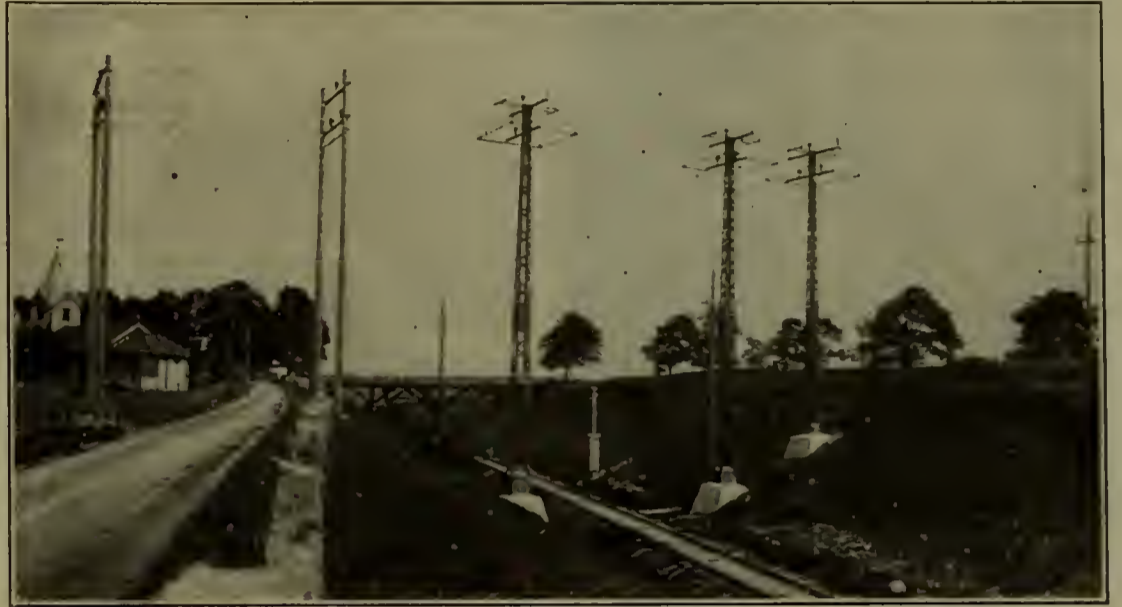
Fig. 17.—50,000-VOLT TRANSMISSION LINE, KYKKELERUD TO HAFSLUND, NORWAY.
