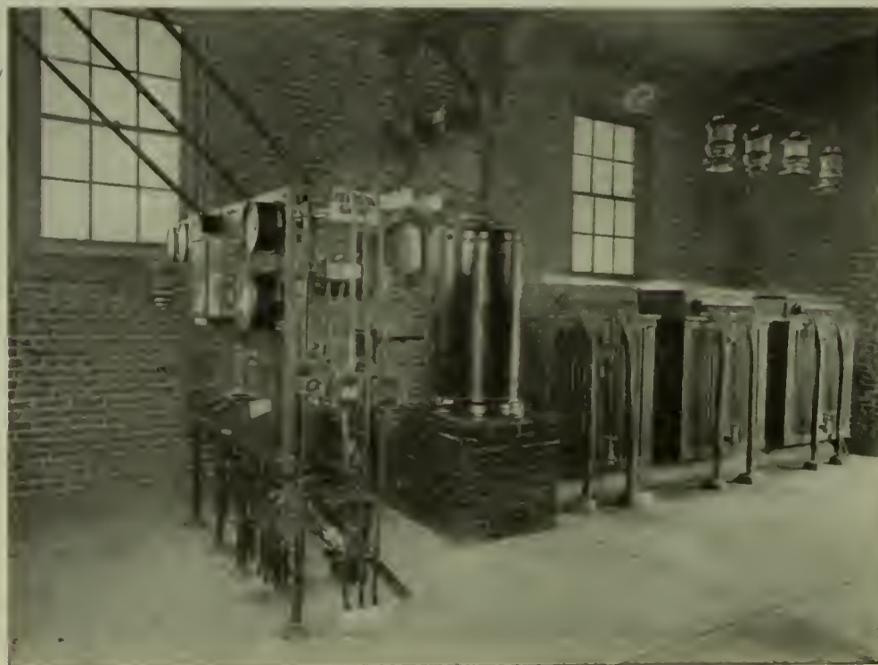
Fig. 12. INTERIOR OF BOULDER SUBSTATION.
