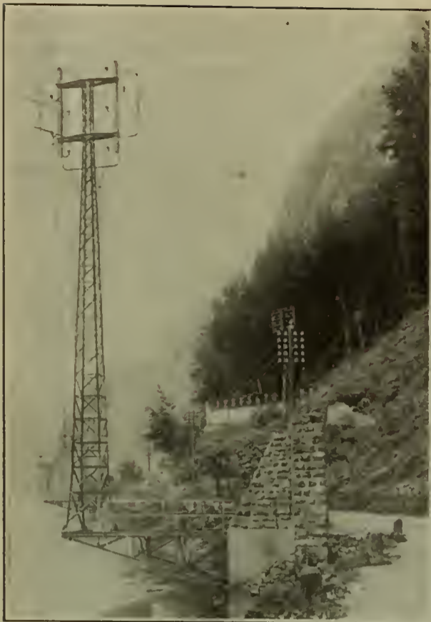
Fig. 19.—27,000-VOLT TRANSMISSION TOWER, OBERMATT-LUCERNE, SWITZERLAND.
