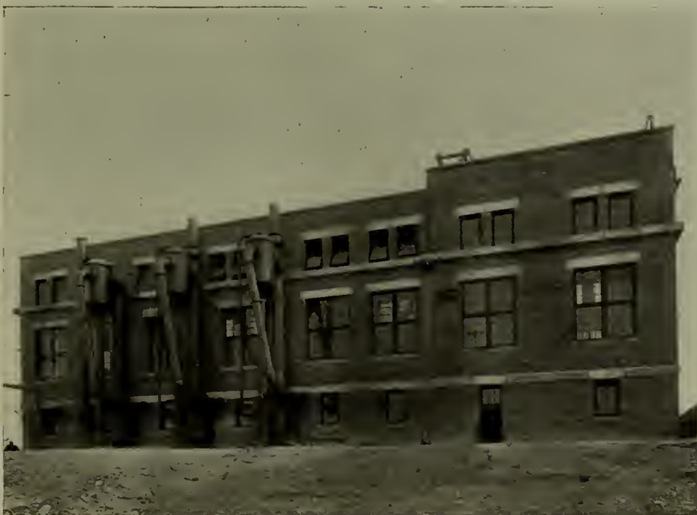
Fig. 3 POWER STATION, RESERVOIR SIDE, SHOWING JET CONDENSERS.
