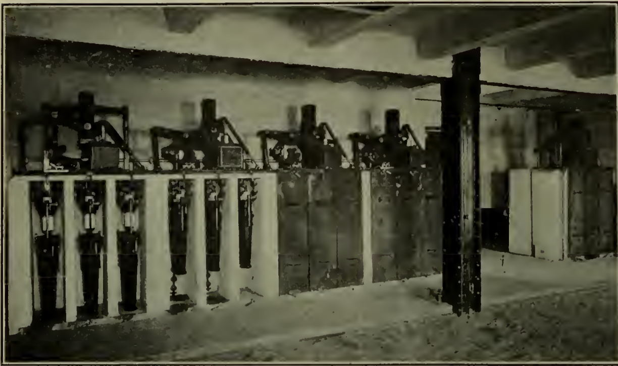
FIG. 5—6600-VOLT LARGE OIL CIRCUIT-BREAKER.
