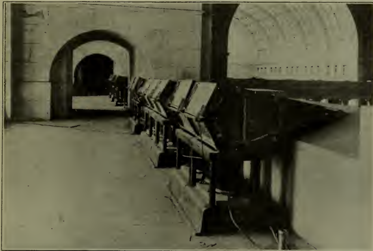
REAR VIEW OF REFLECTOR-FRAMES IN ALCOVE, UNION STATION, WASHINGTON, D. C.
