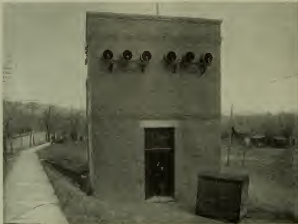
Fig. 11. BOULDER SUBSTATION, 13,000 VOLTS.
