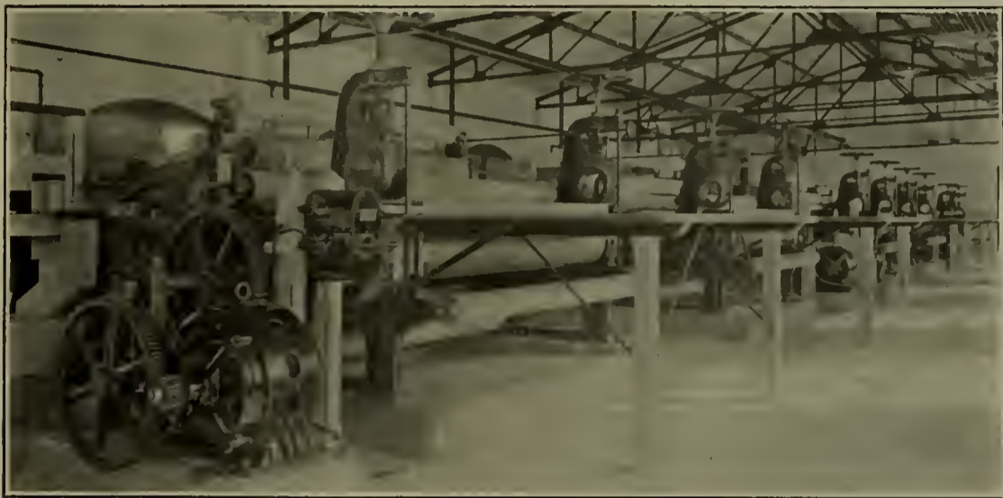
FIG. 3.—FIVE 10-H.P. ALLIS-CHALMERS INDUCTION MOTORS BACK-GEARED TO WET MACHINES.
