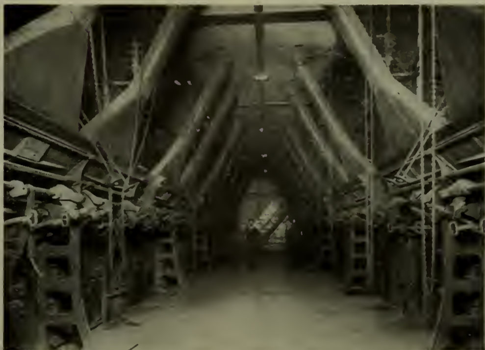
Fig. 8. BOILER ROOM, SHOWING STOKERS AND COAL CHUTES.
