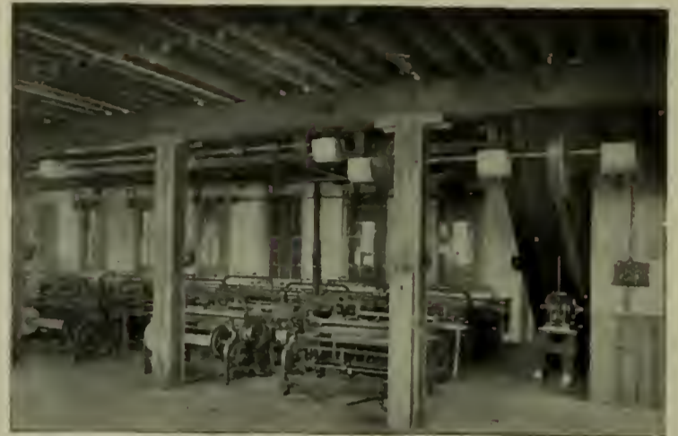
FIG. 4.—10 H.P. 220 VOLT KG SINGLE-PHASE MOTOR IN LOOM ROOM.
