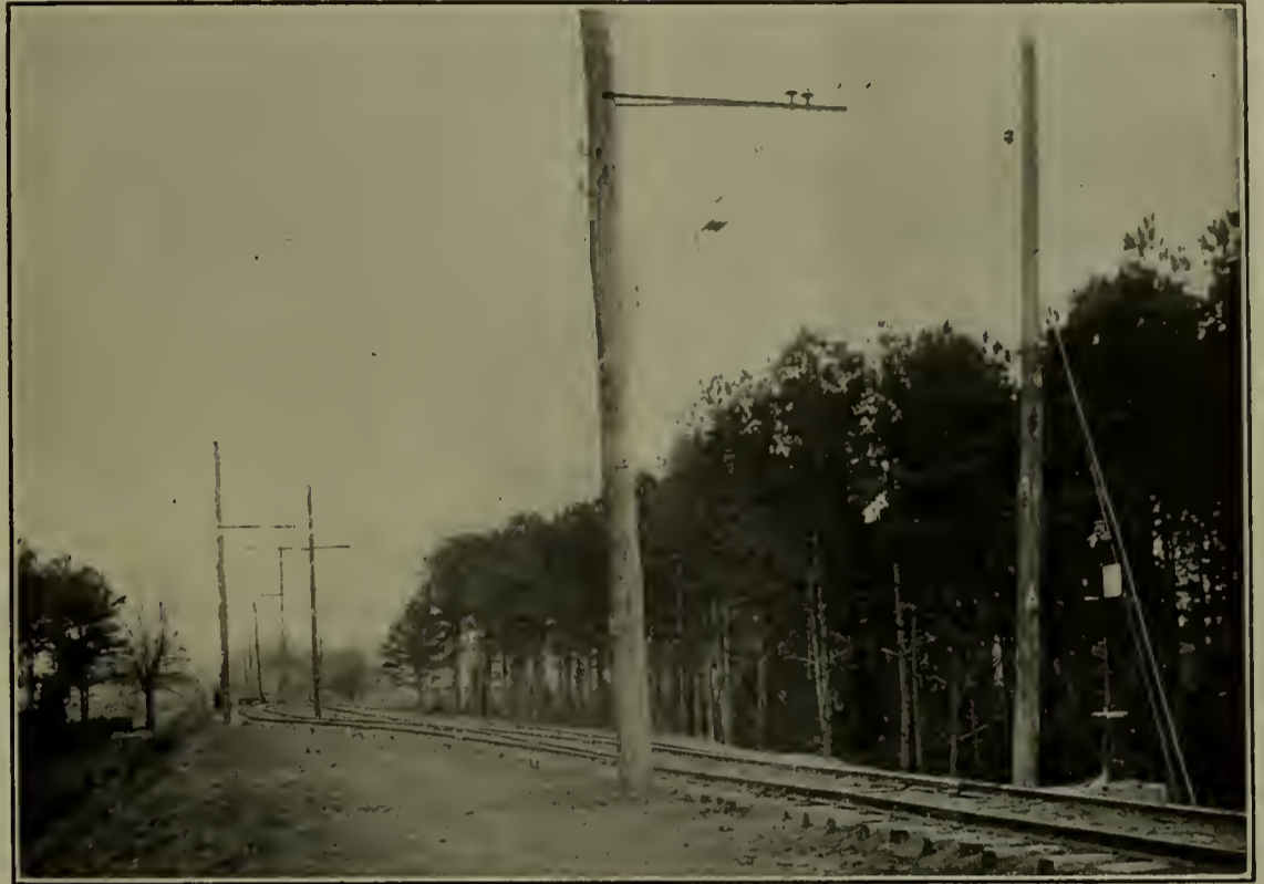
GENERAL VIEW OF TYPICAL TURN-OUT ON RICHMOND & CHESAPEAKE BAY RAILWAY.
