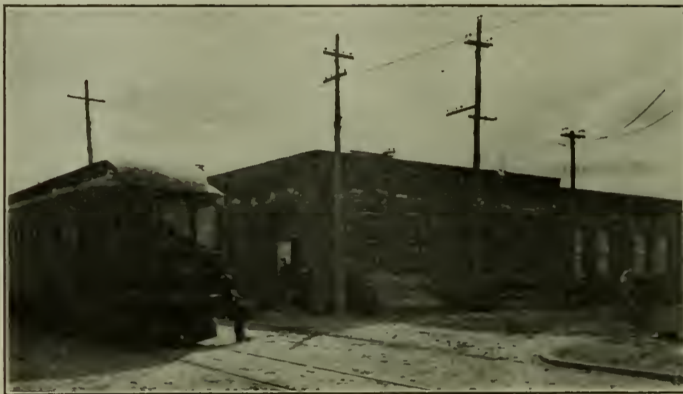
SUBSTATION AT SWAYZEE, IND.
