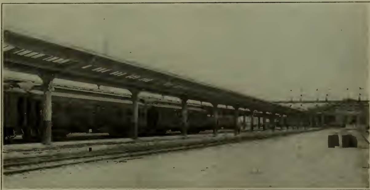
TRAIN SHED LIGHTING, UNION STATION, WASHINGTON, D. C.
