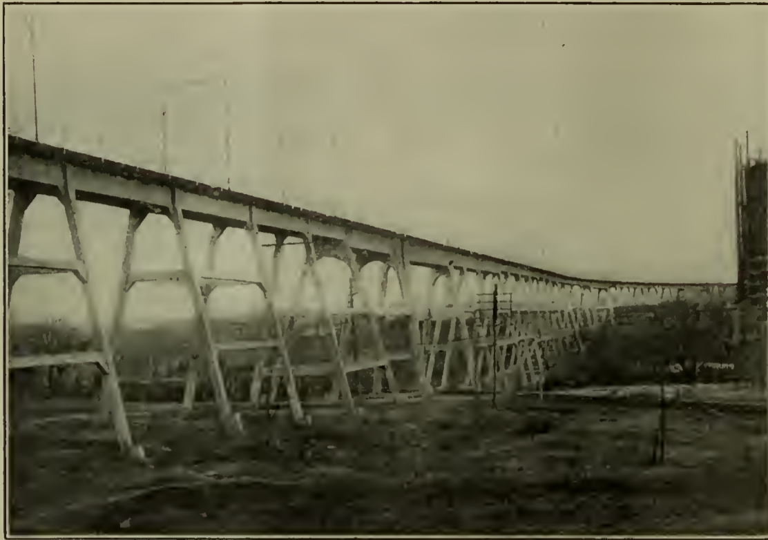
VIEW OF REINFORCED CONCRETE VIADUCT—RICHMOND & CHESAPEAKE BAY RAILWAY.
