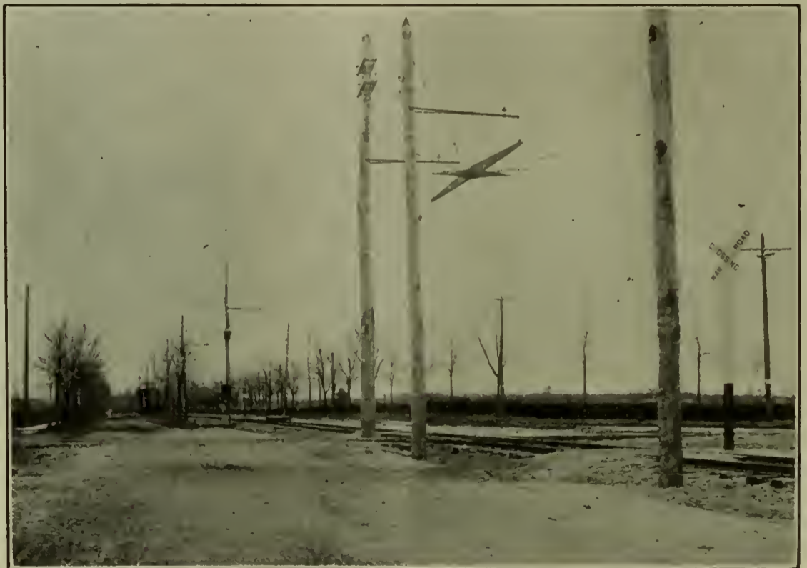
INSULATED CROSS-OVER FOR 600 VOLTS SINGLE PHASE DIRECT CURRENT AND 6600 VOLTS ALTERNATING CURRENT—RICHMOND & CHESAPEAKE BAY RAILWAY.
