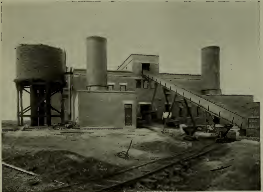
Fig. 2. POWER STATION, BOILER-ROOM SIDE.
