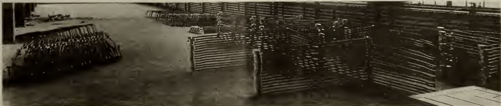
Fig. 7. Conduits bent and fitted ready to be put in place.
