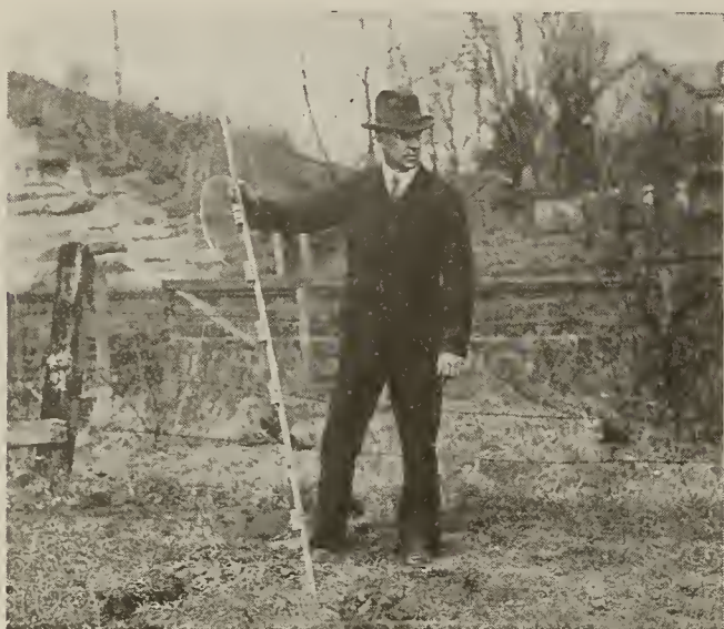
The Charge Ready to be Placed
