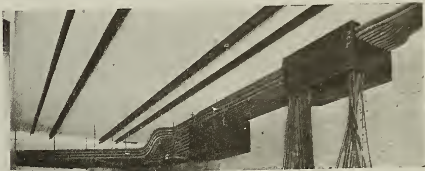
Fig. 6. Neatness of Special Bends
