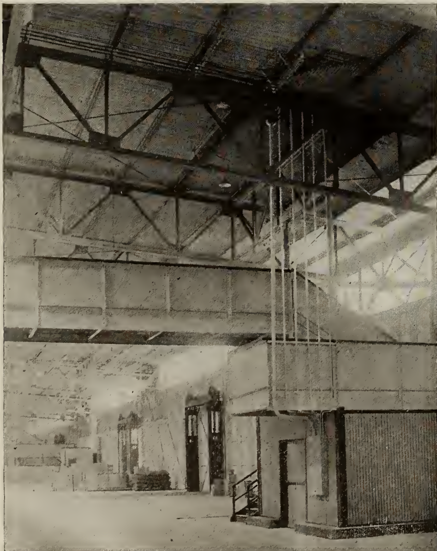
Fig. 1. Interior of Pier
