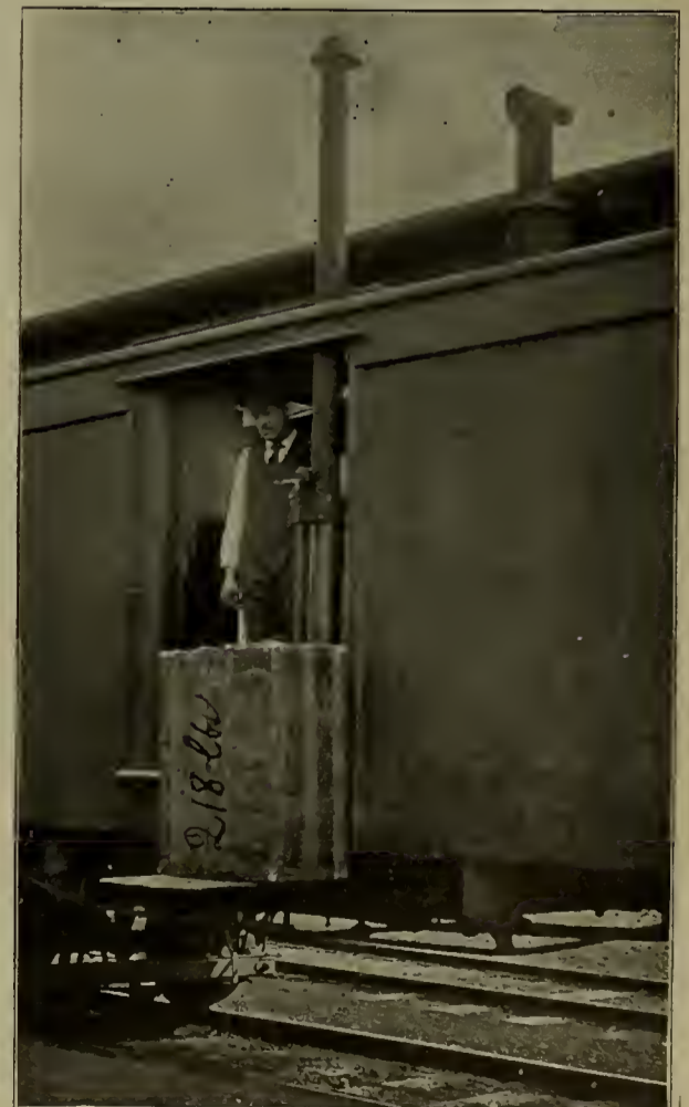
PNEUMATIC BAGGAGE HANDLER.
