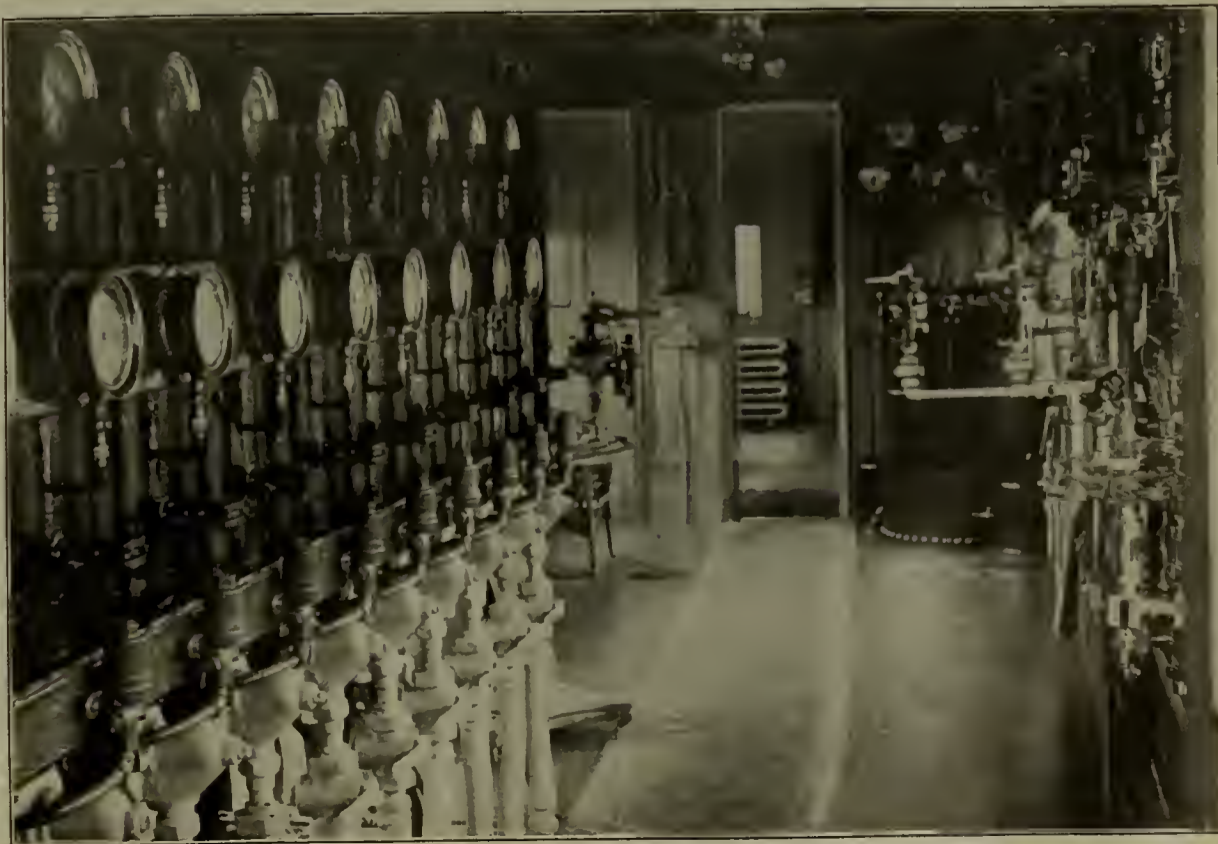
AIR BRAKE INSTRUCTION CAR—N. Y., N. H. & H. RY.—INSTRUCTION ROOM; LOOKING TOWARDS OFFICE.
