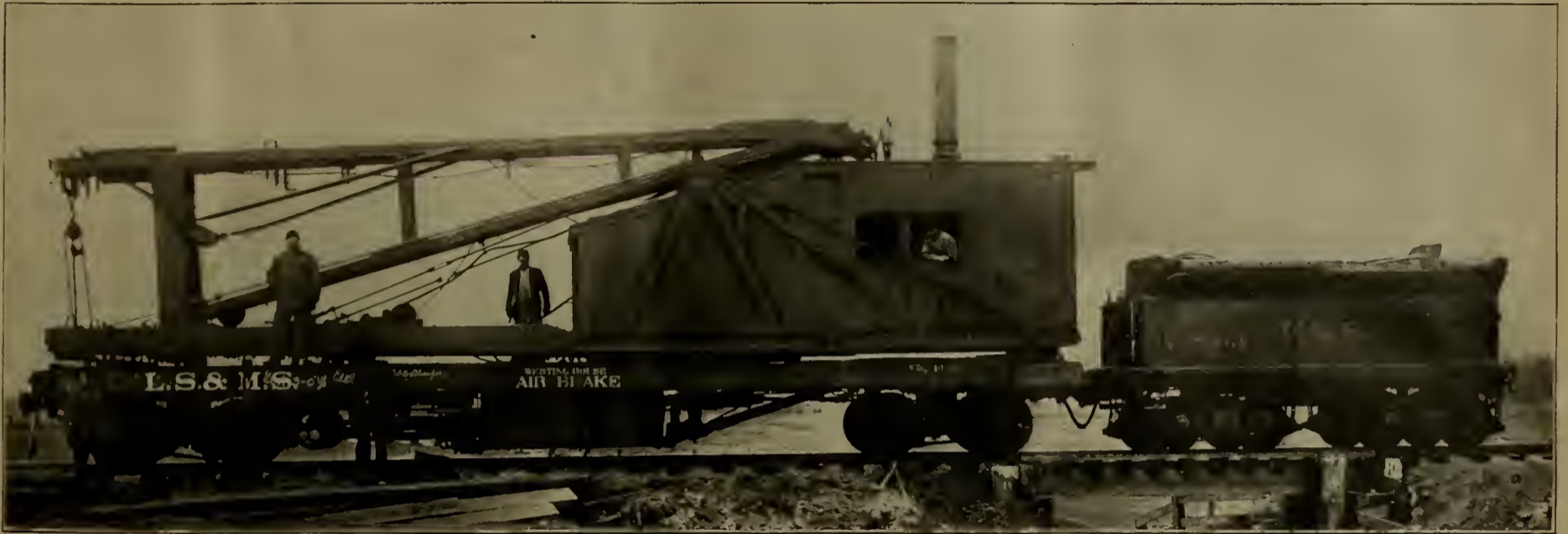
FIG. 1.—PILE DRIVER—L. S. & M. S. RY.—READY FOR THE ROAD.
