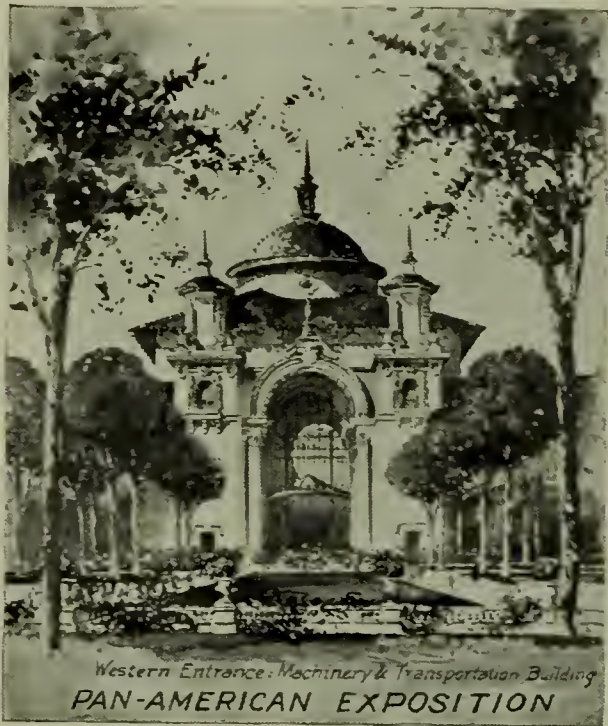
MACHINERY AND TRANSPORTATION BUILDING—WESTERN ENTRANCE.
