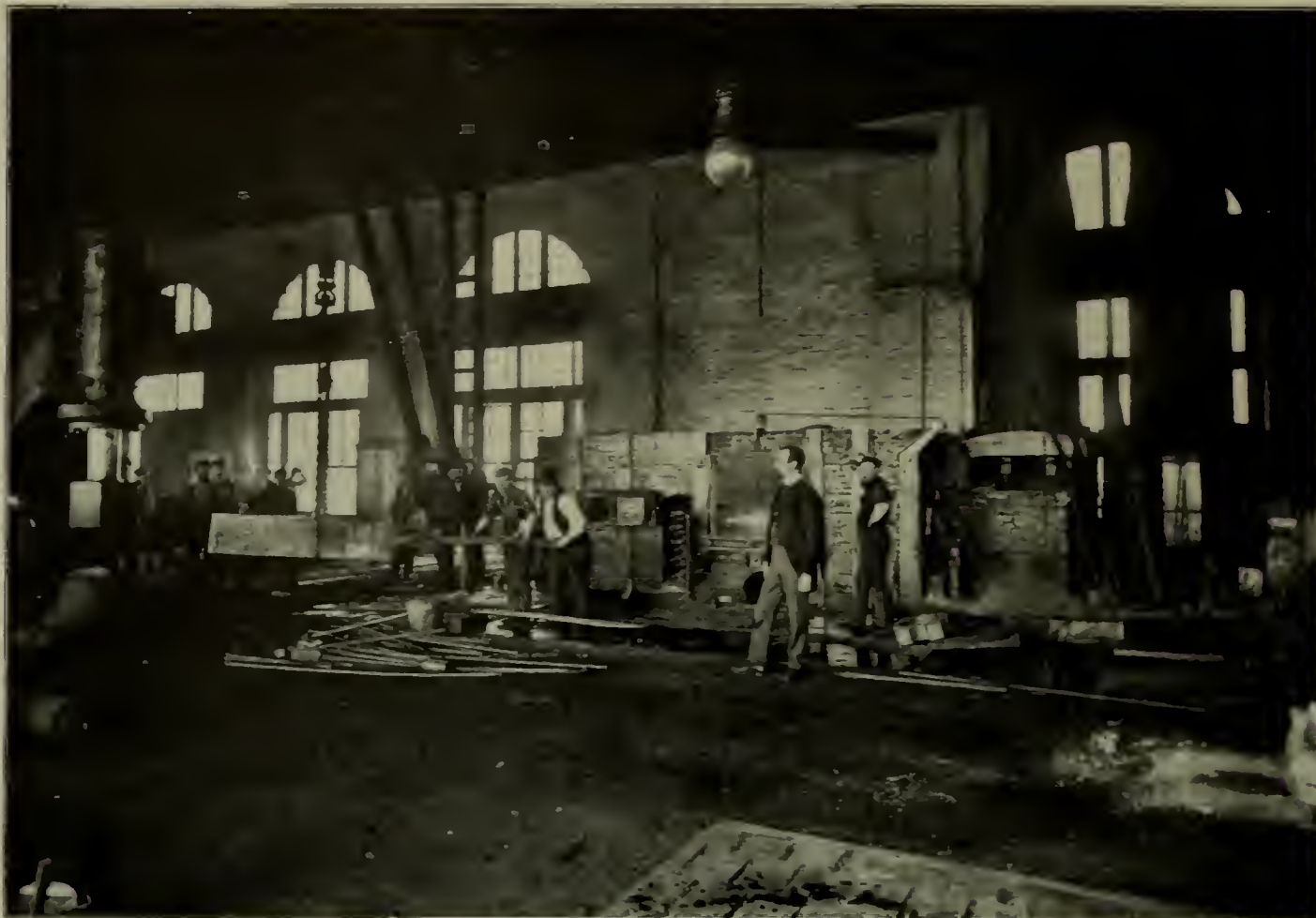
FIGURE 2—WASHINGTON NAVY YARD FORGE SHOP.
