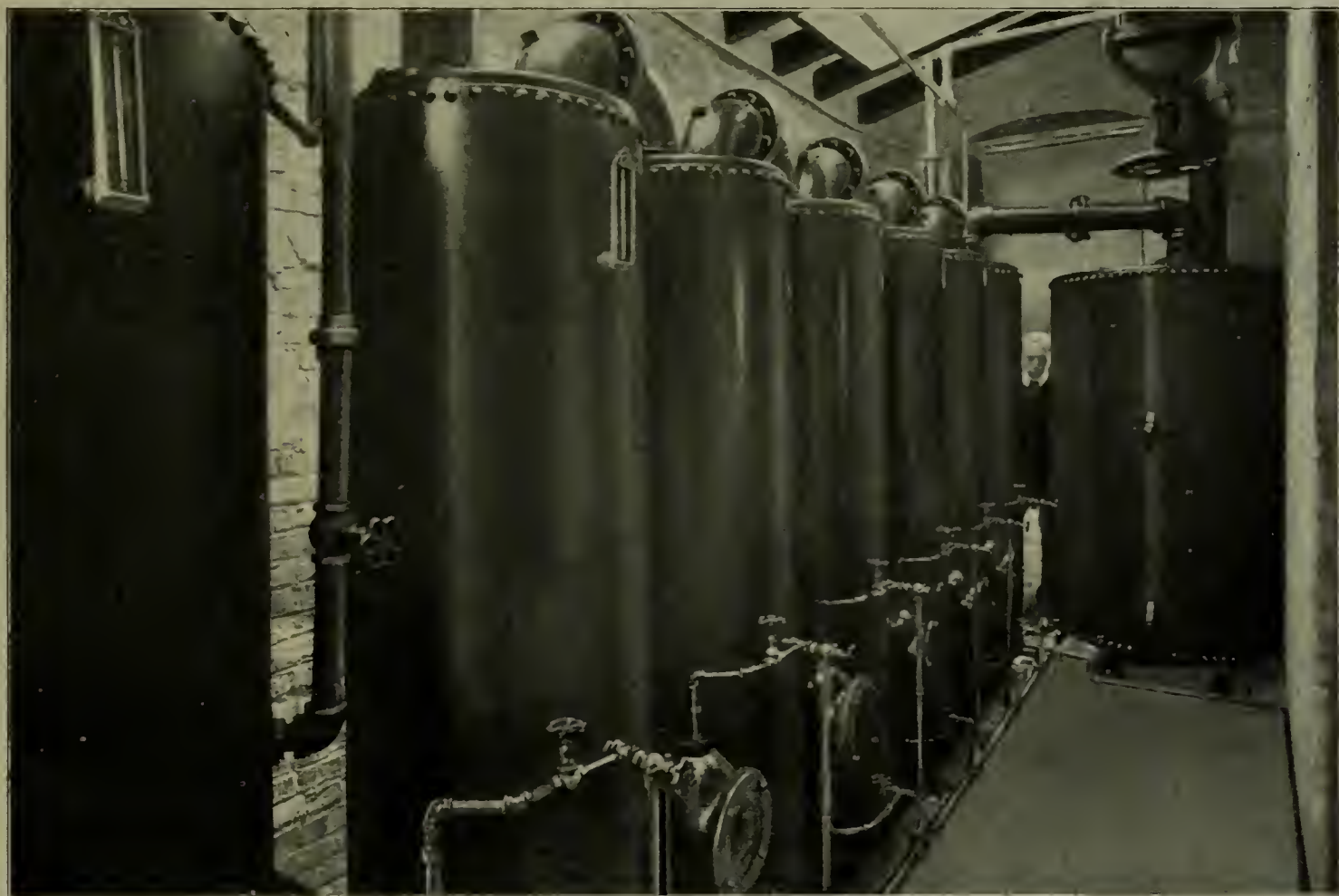
FIGURE 1—TYPICAL SMALL ACME GAS GENERATING PLANT.
