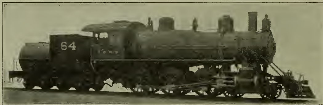
ILLINOIS CENTRAL LOCOMOTIVE WITH VANDERBILT BOILER AND TENDER.
