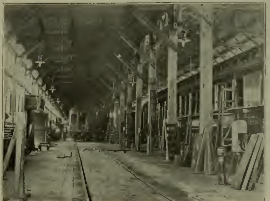
INTERIOR OF CAR REPAIR SHOP SHOWING NORTH BAY—CAR REPAIR SHOPS AT EAST DECATUR, WABASH RAILROAD.
