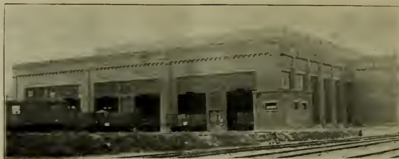
SOUTH END OF FREIGHT CAR REPAIR SHOP, MC KEES ROCKS—PITTSBURGH AND LAKE ERIE R. R. FINISHED CARS LEAVE THIS END.
