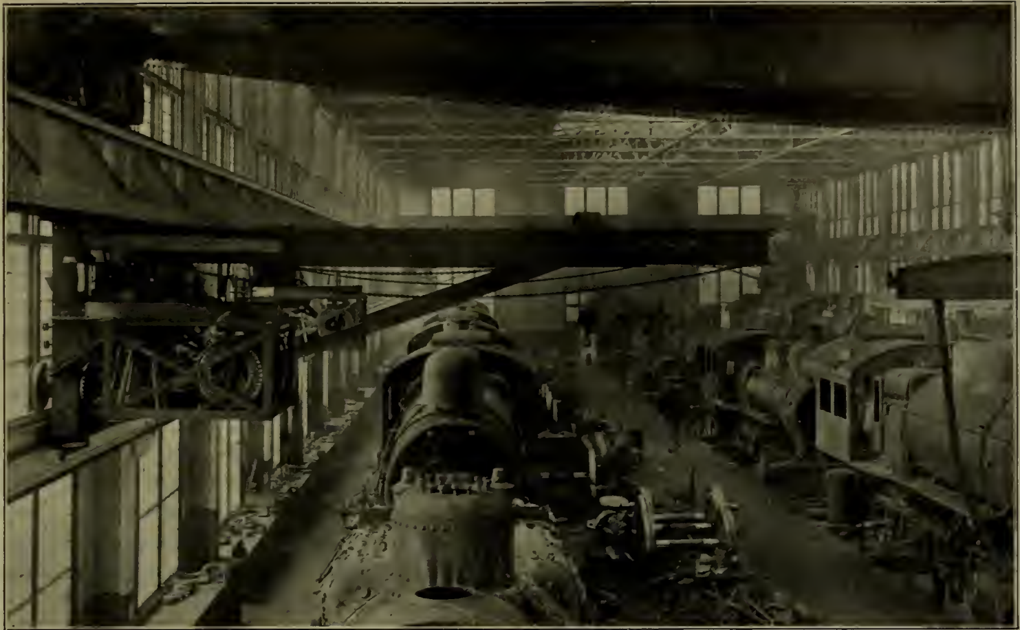
GENERAL ARRANGEMENT OF ERECTING FLOOR SERVED BY HEAVY TRAVELING CRANE, AND WALL CRANES AT ALTOONA SHOPS, — P. R. R.
