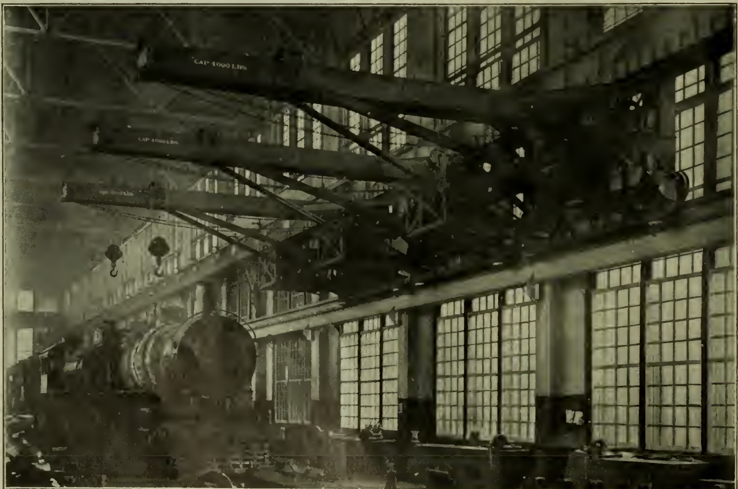
WALL CRANES IN NEW ERECTING SHOP AT ALTOONA—P. R. R.
