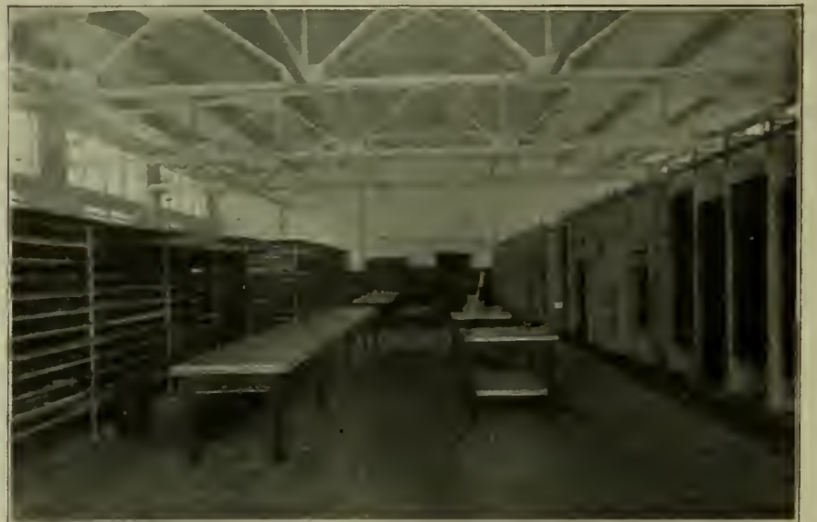
FIG. 3. INTERIOR OF VARNISH ROOM.—KINGSLAND PAINT SHOP, D. L. & W. R. R.
