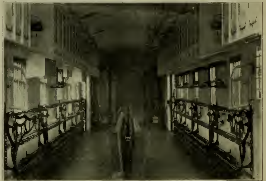
INTERIOR OF ALL STEEL POSTAL CAR, HARRIMAN LINES.
