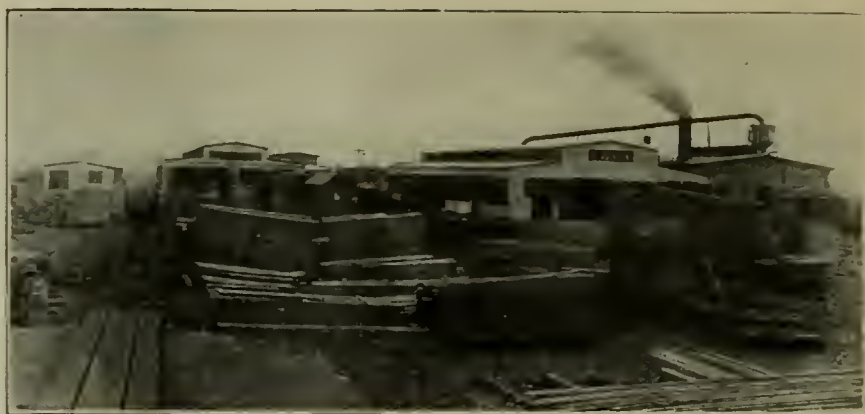
VIEW OF SHOPS FROM NORTHWEST, LUMBER YARD IN FORE GROUND—CAR REPAIR SHOPS AT EAST DECATUR, WABASH RAILROAD.
