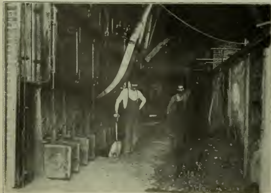
BOILER ROOM SHOWING DELIVERY TUBES FOR SHAVINGS—CAR REPAIR SHOPS AT EAST DECATUR, WABASH RAILROAD.
