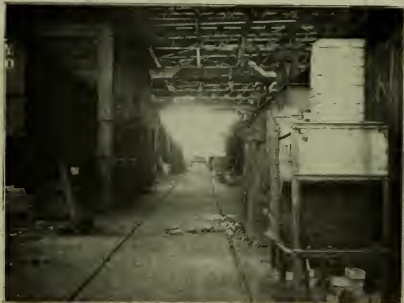
INDUSTRIAL TRACK THROUGH CENTER OF STEEL CAR BAY. RIVET FURNACE ON RIGHT, STEEL CAR JACK ON LEFT—FREIGHT CAR REPAIR SHOP, MC KEES ROCKS, PITTSBURGH AND LAKE ERIE R. R.
