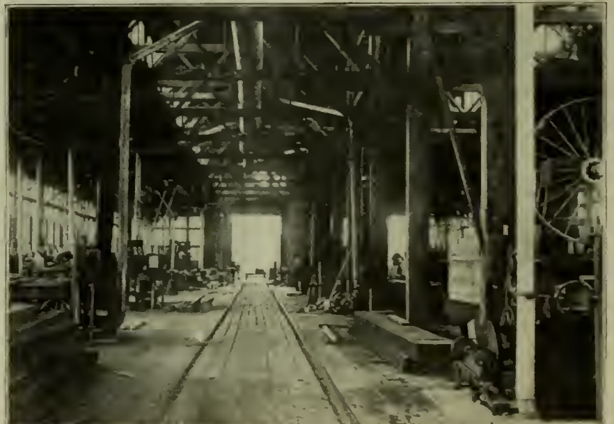
VIEW DOWN MATERIAL TRACK IN NORTH BAY OF PLANING MILL—CAR REPAIR SHOPS AT EAST DECATUR, WABASH RAILROAD.
