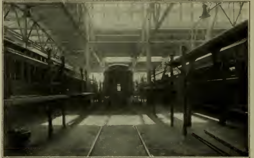
FIG. 2. INTERIOR OF KINGSLAND PAINT SHOP, D. L. & W. R. R., SHOWING TYPE OF SCAFFOLDS USED.
