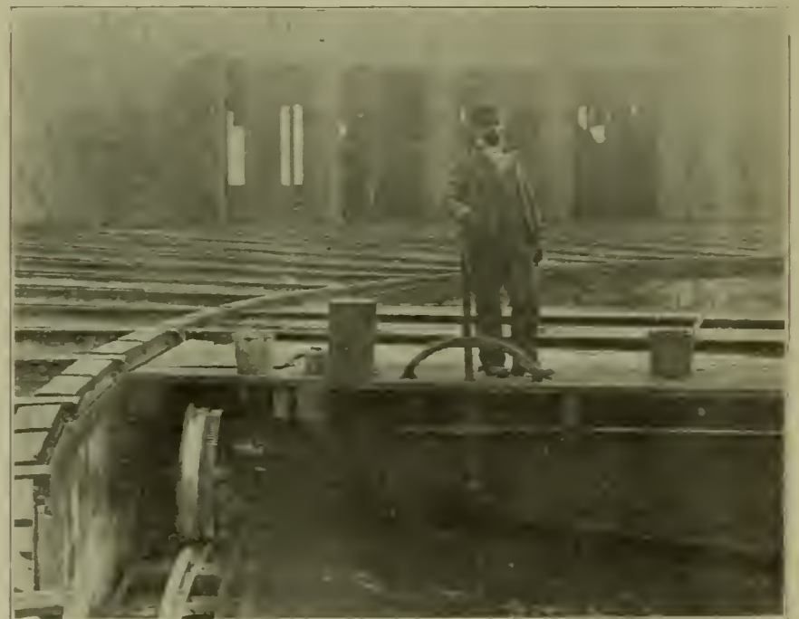
TURNTABLE DRIVEN BY J. L. PILLING AIR MOTOR. OPERATING LEVER IS SHOWN. ANOTHER LEVER IS PLACED AT THE OTHER END OF THE TABLE SO TABLE CAN BE OPERATED FROM EITHER END—LOCOMOTIVE TERMINAL AT CHICAGO, C. & W. I. R. R.
