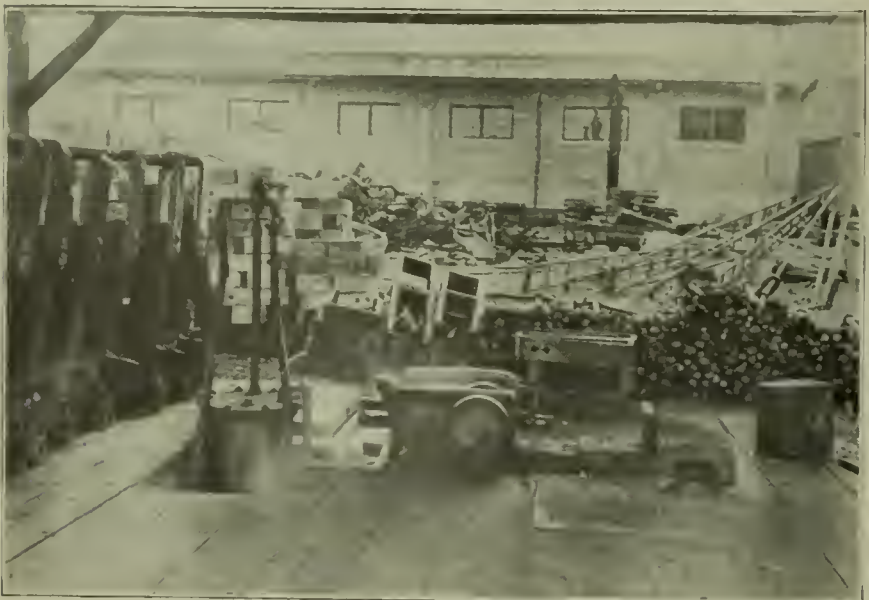
COUPLER YOKE RIVETING PRESS, LOCATED UNDER SHED, WEST OF BLACKSMITH SHOP—CAR REPAIR SHOPS AT EAST DECATUR, WABASH RAILROAD.
