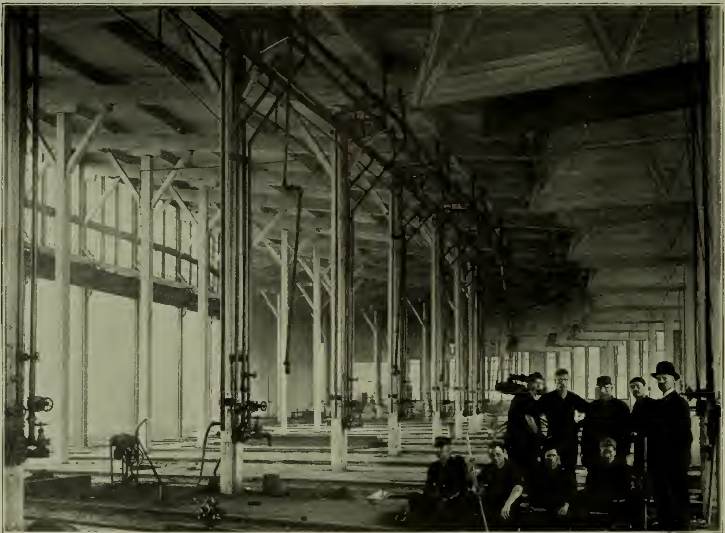
INTERIOR OF 49TH ST. ROUNDHOUSE OF THE CHICAGO & WESTERN INDIANA R. R., SHOWING ARRANGEMENT OF CONNECTIONS OF THE MILLER SYSTEM.
