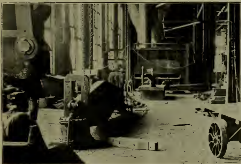
VIEW IN MACHINE SHOP ADJACENT TO STEEL CAR BAY. RIVETER AND ANGLE PRESS IN FOREGROUND WITH STRAIGHTENING TABLE AND FURNACE BEYOND.—FREIGHT CAR REPAIR SHOP, MC KEES ROCKS, PITTSBURGH AND LAKE ERIE R. R.
