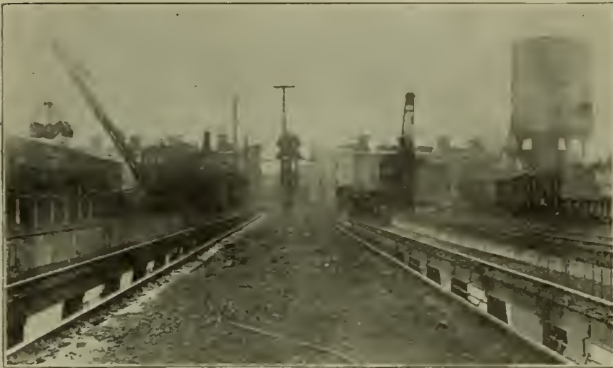
VIEW SHOWS THE TWO CINDER PITS. IN THE BACKGROUND ARE THE TWO LOCOMOTIVE CRANES. ON THE LEFT COAL STORAGE BINS, ON THE RIGHT COAL CARS FOR LOADING DIRECT TO THE LOCOMOTIVE TENDERS—LOCOMOTIVE TERMINAL AT CHICAGO, C. & W. I. R. R.
