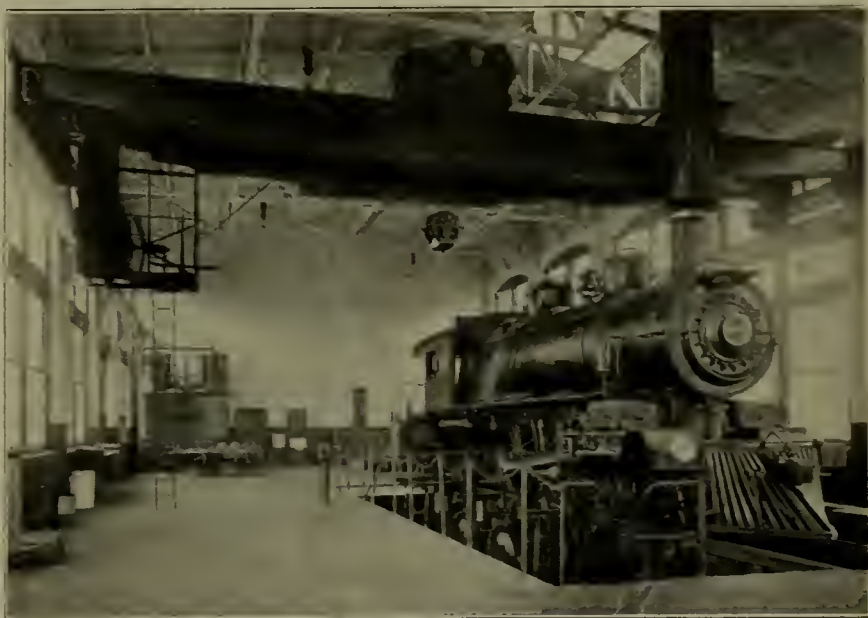
INTERIOR OF LOCOMOTIVE TESTING PLANT AT ALTOONA, SHOWING LOCOMOTIVE IN POSITION FOR TEST—PENNSYLVANIA R. R.
