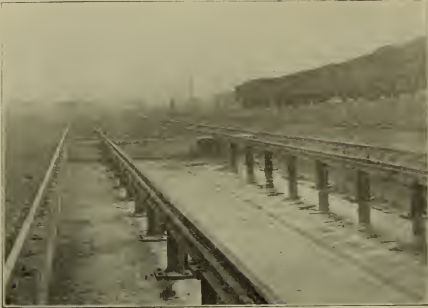
INSPECTION PIT—LOCOMOTIVE TERMINAL AT CHICAGO, C. & W. I. R. R.
