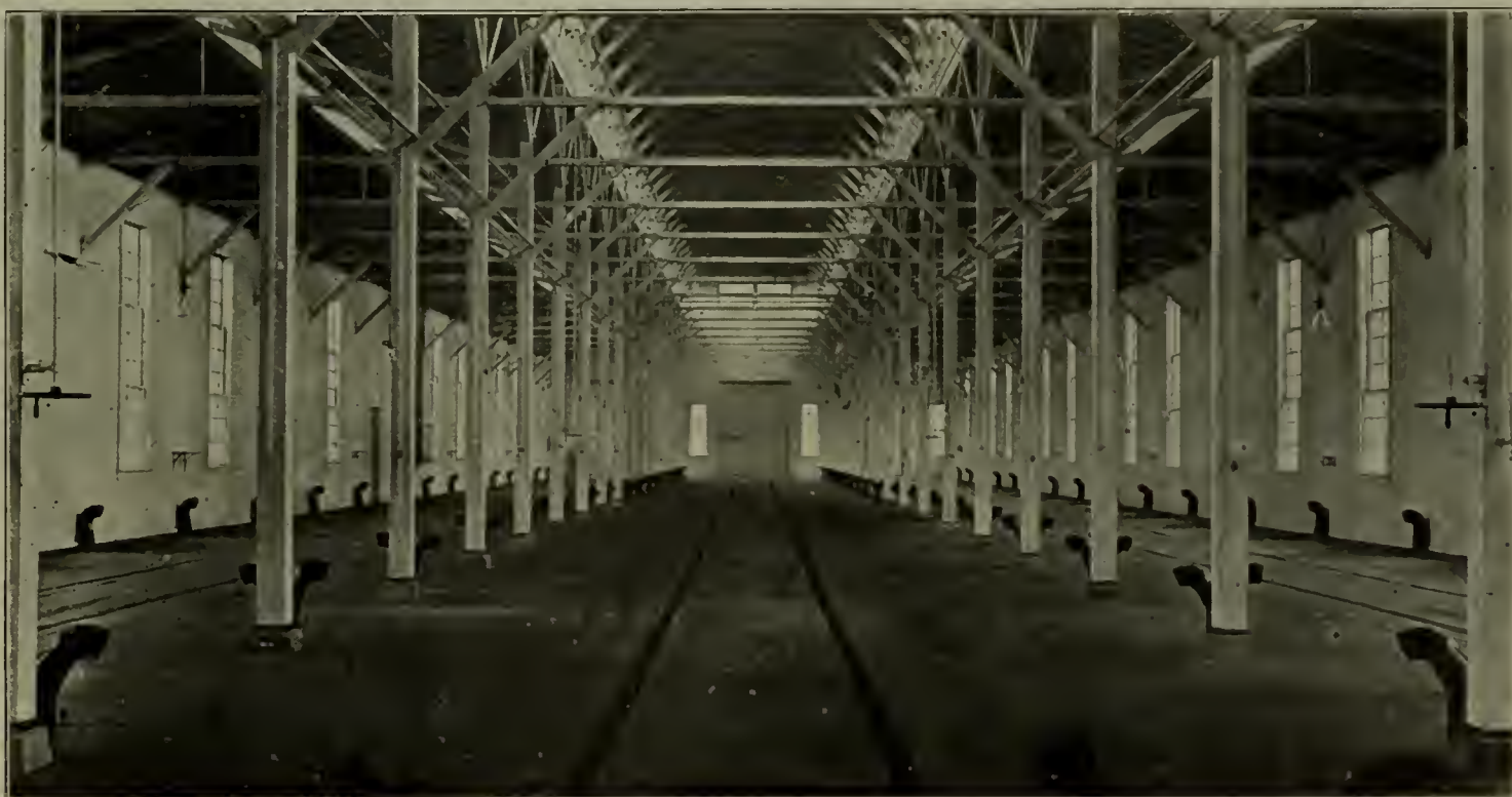
INTERIOR OF PAINT SHOP SHOWING ARRANGEMENT OF OUTLETS FOR HEATING SYSTEM--NEW PAINT SHOP AT MIDDLETOWN, N. Y. O. & W. RY.
