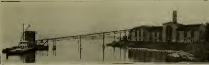
POWER HOUSE AND COAL UNLOADING STATION AND CONVEYOR AT COS COB, CONN., THE MAIN GENERATING STATION FOR THE ELECTRIFIED LINES OF THE NEW YORK, NEW HAVEN & HARTFORD R. R. OUT OF NEW YORK CITY.
