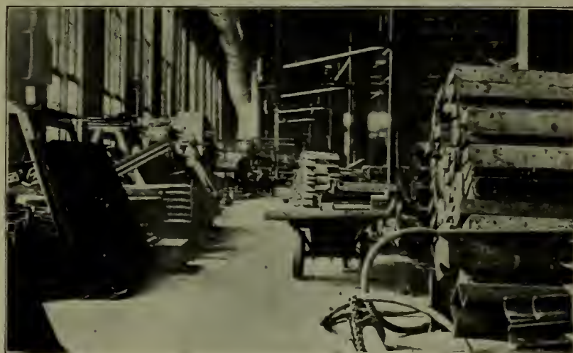
STORAGE ROOM FOR STEEL REPAIR PARTS, OVERHEAD TROLLEY CRANE IS SHOWN AND TRUCK FOR HANDLING PARTS.—FREIGHT CAR REPAIR SHOP, MC KEES ROCKS, PITTSBURGH AND LAKE ERIE R. R.
