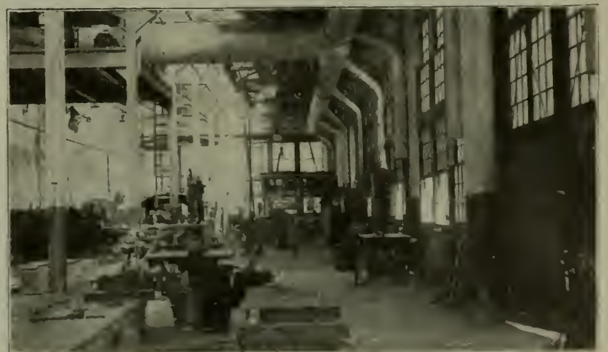
INTERIOR OF WOOD WORKING SHOP—LOCOMOTIVE SHOPS AT TRENTON, PENNSYLVANIA R. R.
