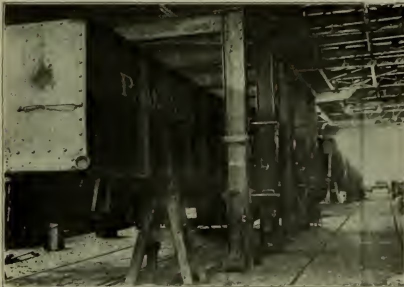
VIEW OF STEEL CAR REPAIR JACK FOR STRAIGHTENING UP STEEL CAR BODIES—FREIGHT CAR REPAIR SHOP, MC KEES ROCKS, PITTSBURGH AND LAKE ERIE R. R.
