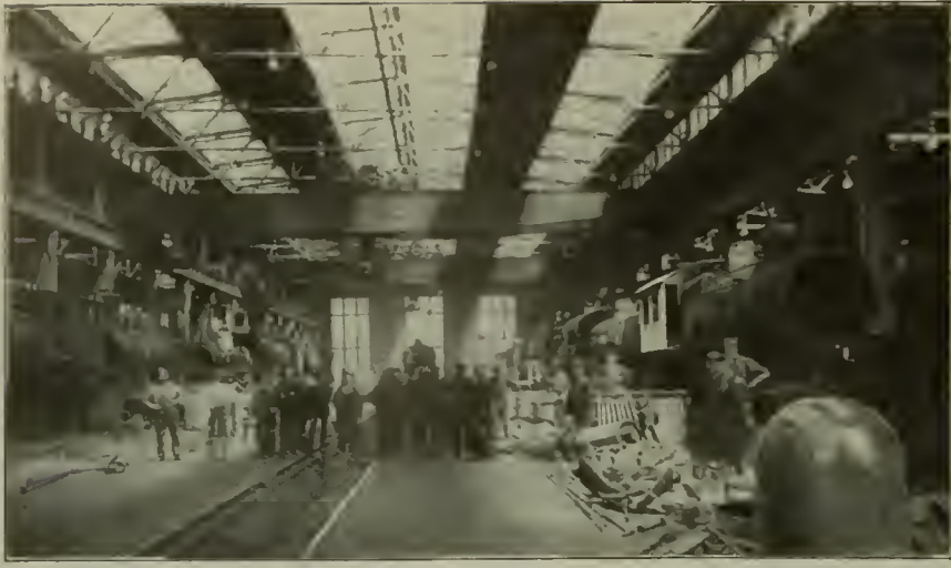
INTERIOR OF ERECTING SHOP—LOCOMOTIVE SHOPS AT TRENTON, PENNSYLVANIA, R. R.
