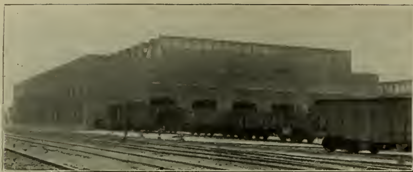
NORTH END OF FREIGHT CAR REPAIR SHOP, MC KEES ROCKS—PITTSBURGH AND LAKE ERIE R. R.—BAD ORDER CARS ENTER THE SHOP FROM THIS END.
