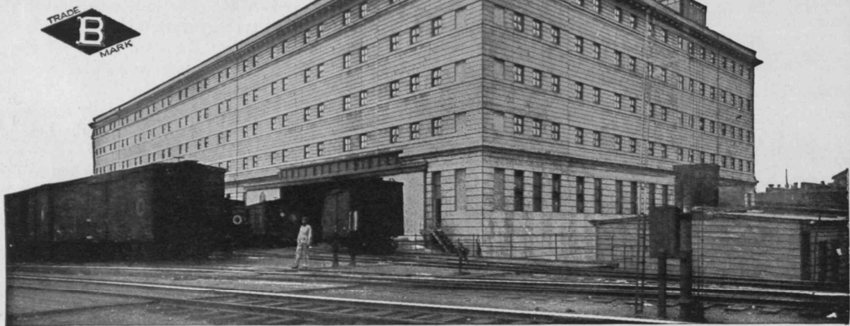
Designed and constructed by John W. Ferguson Co., Paterson, N. J., under the general supervision of Joseph O. Osgood, Chief Engineer of the Central R. R. of N. J.
