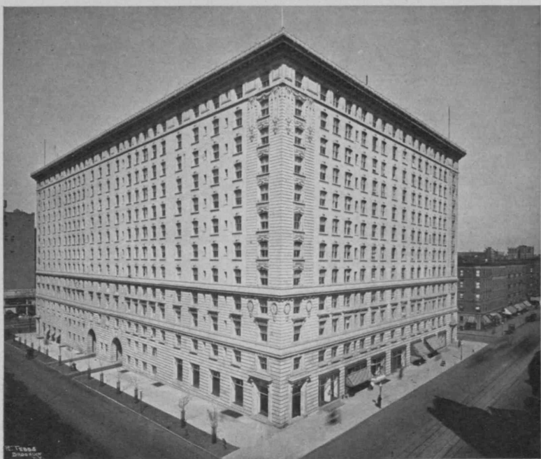
The Belnord Apartments H. Hobart Weeks, Archt. 86th St. and Broadway, New York Largest Apartment-House in the World Brick and Gray Atlantic Terra Cotta
