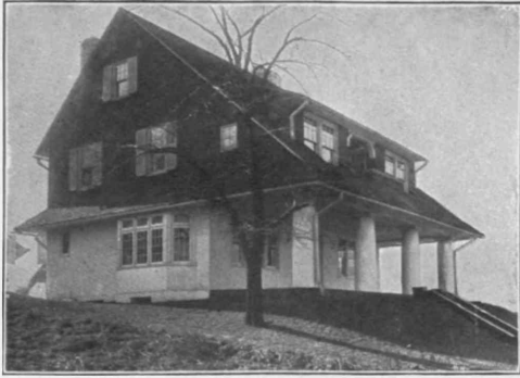
Stained with Cabot's Shingle Stains & Water-proof Cement Stains RUFUS D. WOOD, Architect, Pittsburgh
