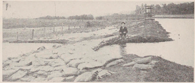
SANDBAGGING THE RIVER
