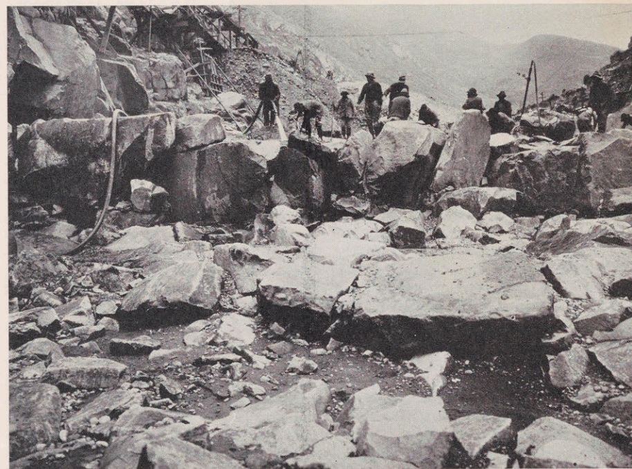
WASHING FINES INTO VOIDS
