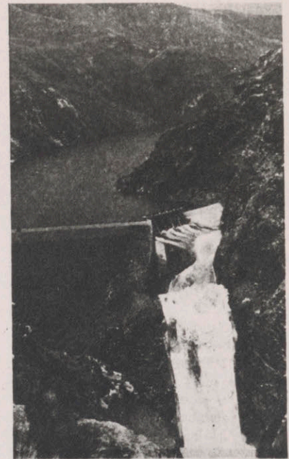
Malpaso dam passing 4500 second feet of water.
