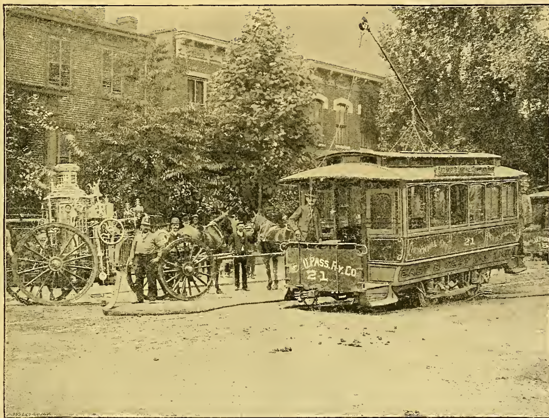
METHOD OF JUMPING FIRE HOSE ON TRACK ON RICHMOND, VA., ROAD.
