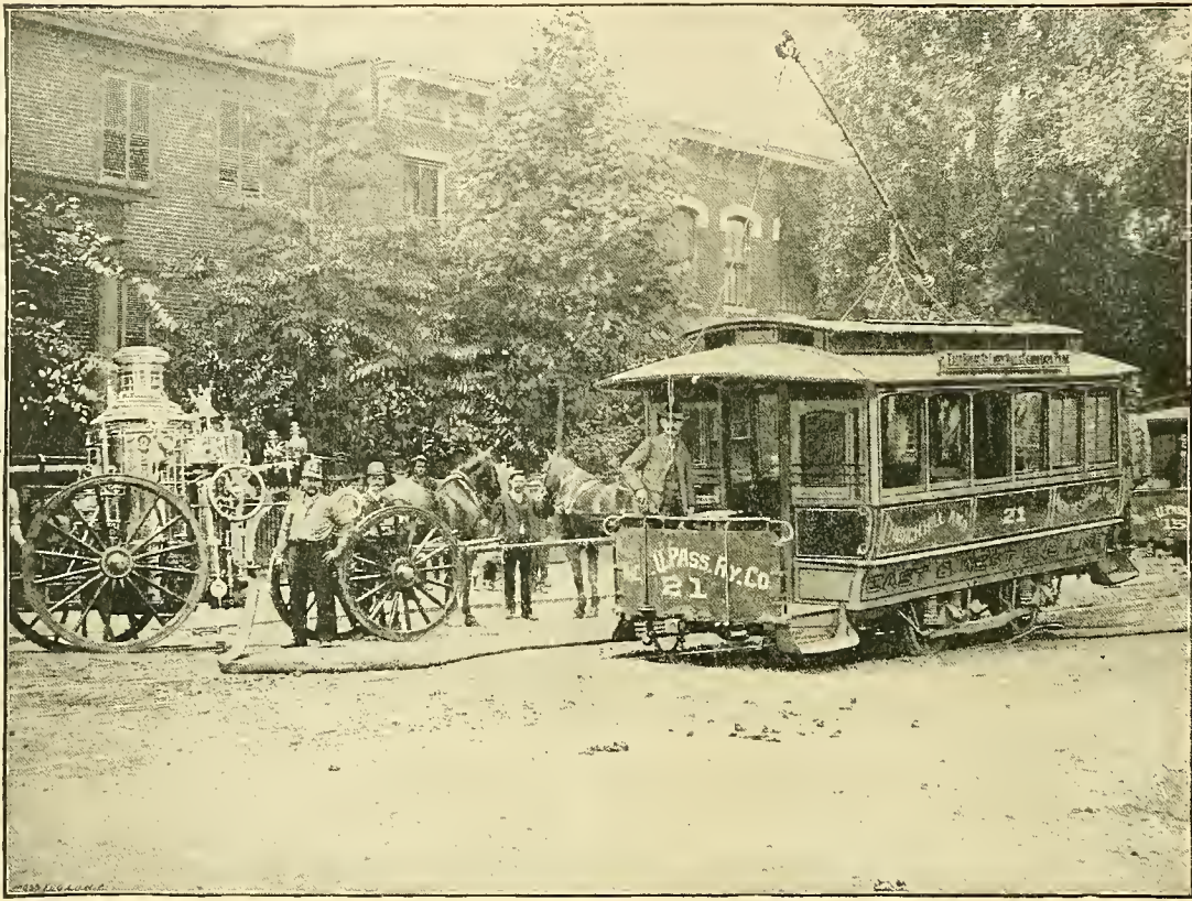
METHOD OF CROSSING FIRE HOSE IN RICHMOND, VA.—CAR JUMPING FIRE HOSE.
