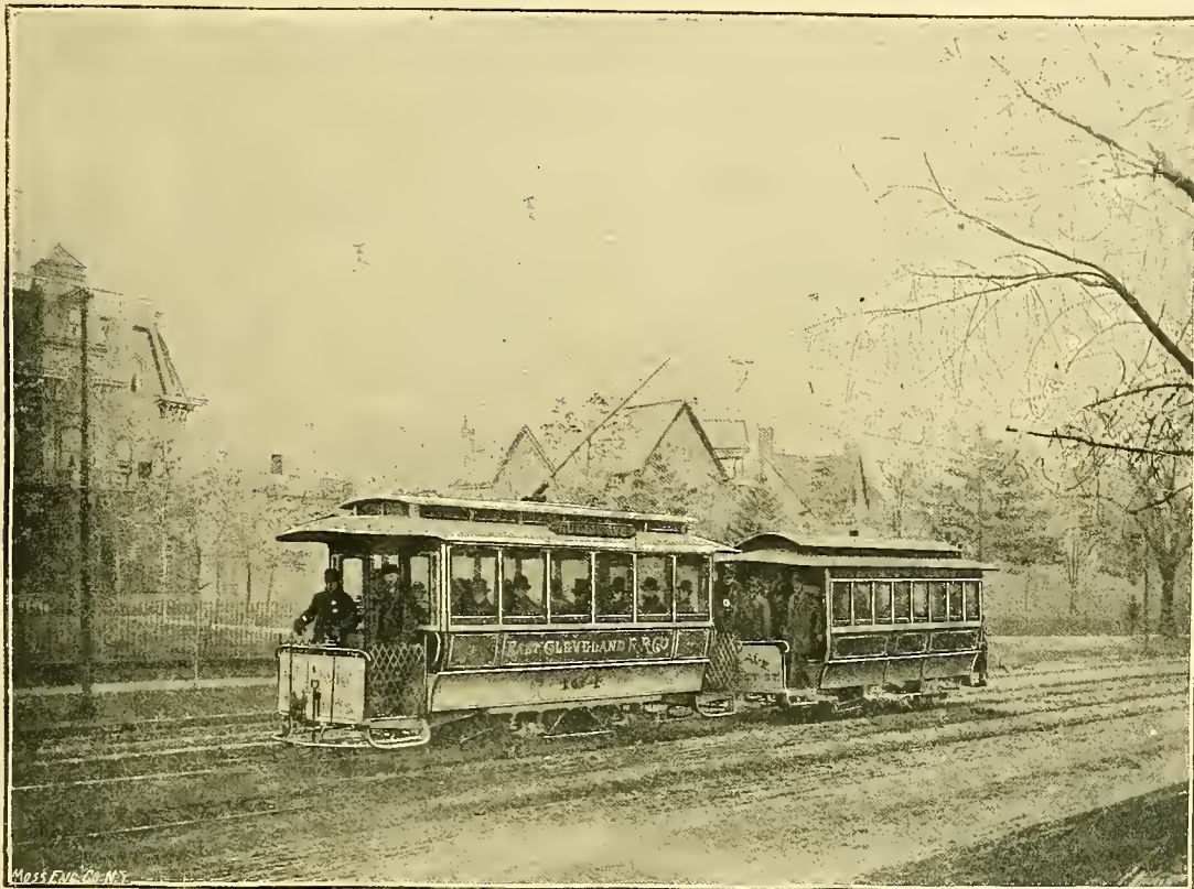
EAST CLEVELAND R. R. Co.—ELECTRIC DIVISION.
