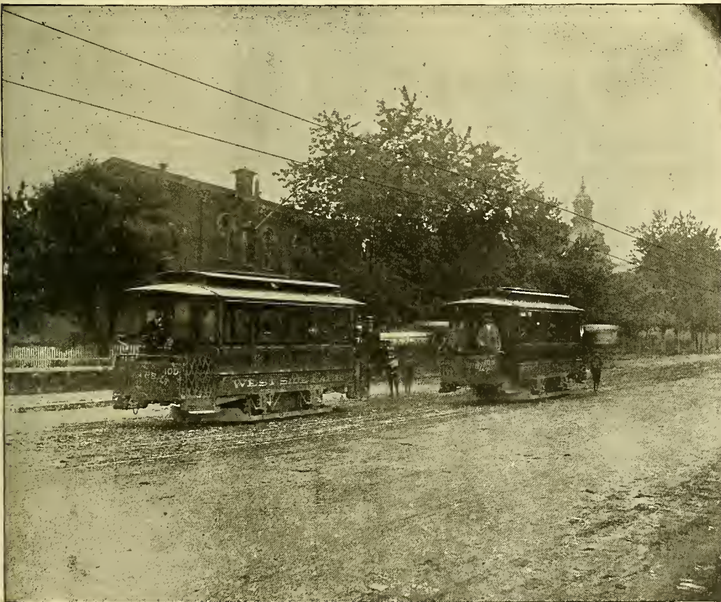
McGAVOCK & MT. VERNON ELECTRIC RAILWAY, NASHVILLE, TENN.
